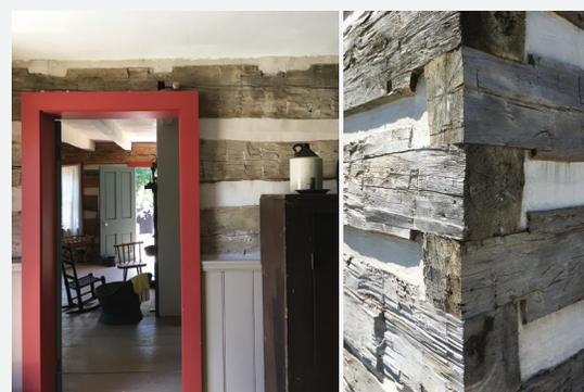
Above Left: Interior of the Pendergast Log House with traditional colour scheme and limewash finish on the walls and ceiling. Above Right: The log house's original structure was concealed for years by a brick veneer applied sometime in the 1920s. The brick cladding helped protect it for almost a century.
