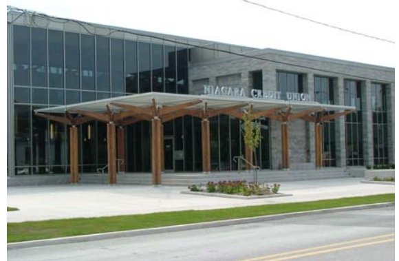
Canopy over building entrance
