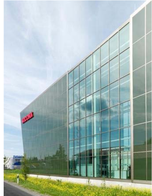
Architecture with a high window-to-wall ratio
