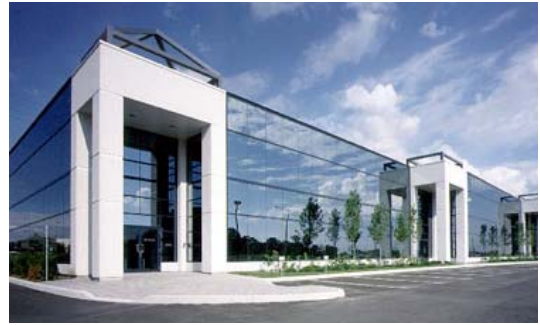
Vehicular Access to Building
