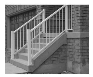
Figure 3.5a: Acceptible Precast Step Solution
