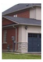
Figure 8.15.2: Example of Unnacceptable Material Transition
