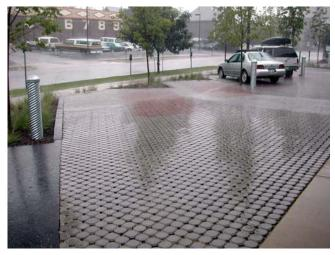
Figure 2.1 - Permeable Paving
