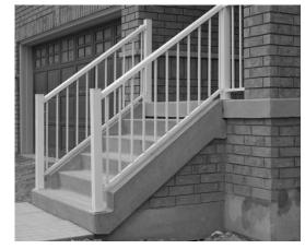
Figure 8.15.4b: Acceptable Precast Step Solution
