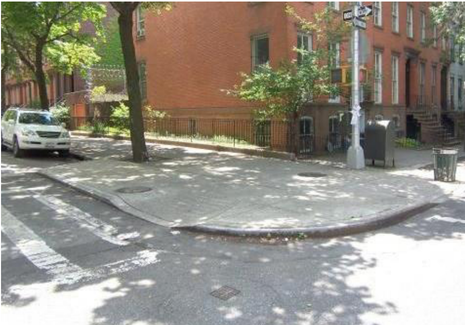
Sidewalk extension: shortens crossing distance, slows turning cars
