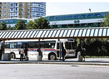
Downtown Brampton Terminal
