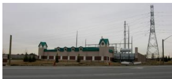
Jim Yarrow Municipal Transfer Station
