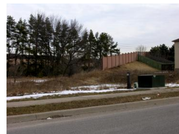
Residential Rail Noise Wall— Ravenscliffe Court
