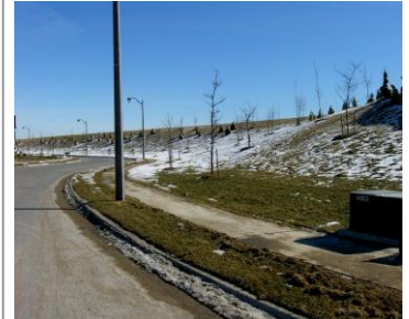
Torbram Road Noise Berm
