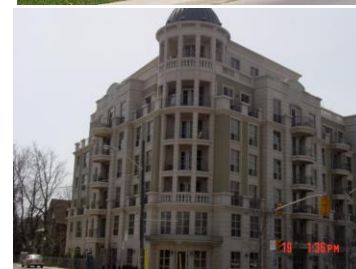
Examples of Mid-Rise Building
