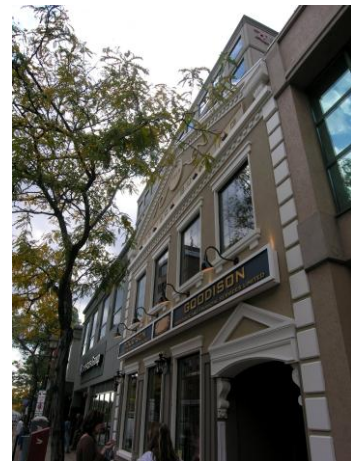
Building Façade Improvements
