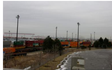
Brampton CN Intermodal Terminal
