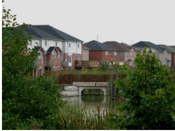
McClure Channel – Opportunity for Stormwater Recharge
