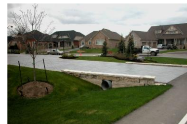
Springbrook Surface Run-off Treatment
