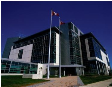
Grenville & William Davis Courthouse
