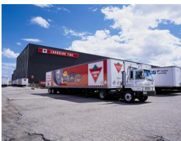
Canadian Tire Warehouse
