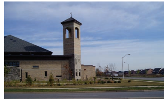
Figure 7.0b - Architectural element at corner location
