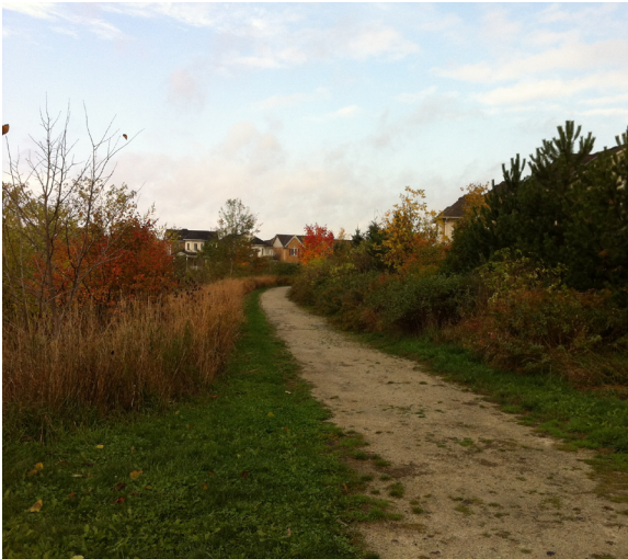
Fig. 3.3.2e - For local trail loops within the green system trails, preference shall be given to using materials that are permeable and require minimal maintenance, such as screenings.
