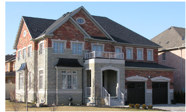
Fig 3.4.4b: High quality detailing is required on both street facing facades of a corner lot dwelling unit
