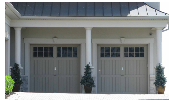
Fig.3.4.3p: High quality of materials should be adopted for driveways and garage doors
