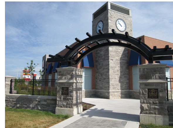
Fig. 3.1.2.6c - Image example of how the gateway material and design theme can reflect or be complementary to the adjacent built form.
