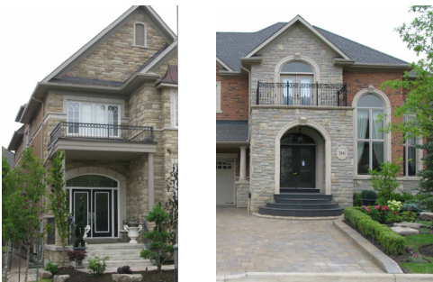
Fig 3.4.4d: Balconies above porches are highly encouraged on Community Gateway and Community Window Street Lots
