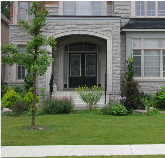
Fig.3.4.3d: Door glazing should be provided to allow for natural light in the dwelling's main foyer
