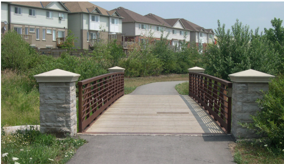
Fig. 3.3.2f - Image example of a pedestrian bridge crossing with standard prefabricated steel structure and wood decking, with an upgraded masonry/stone column component.
