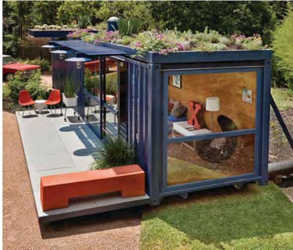
Flat Green Roof Precedent (by Poteet Architects)
