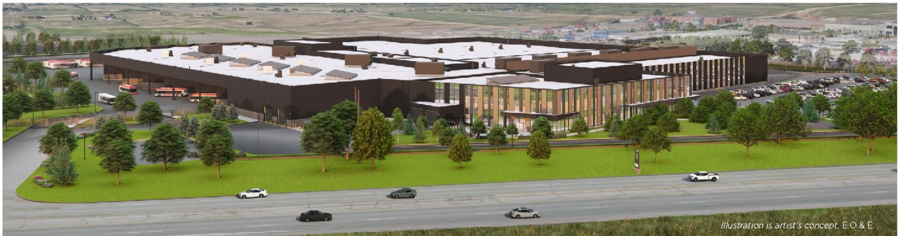
Construction of Third Transit Facility
