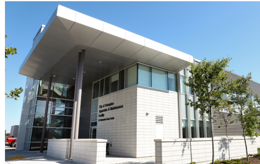
Fig 4.6.2 Brampton Apparatus and Maintenance Facility Entrance
