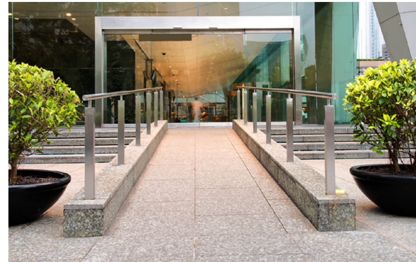
Fig 4.6.1 High Rise Accessible Entrance
