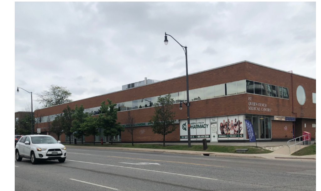
Fig 2.1.6 Office Building Along Centre Street
