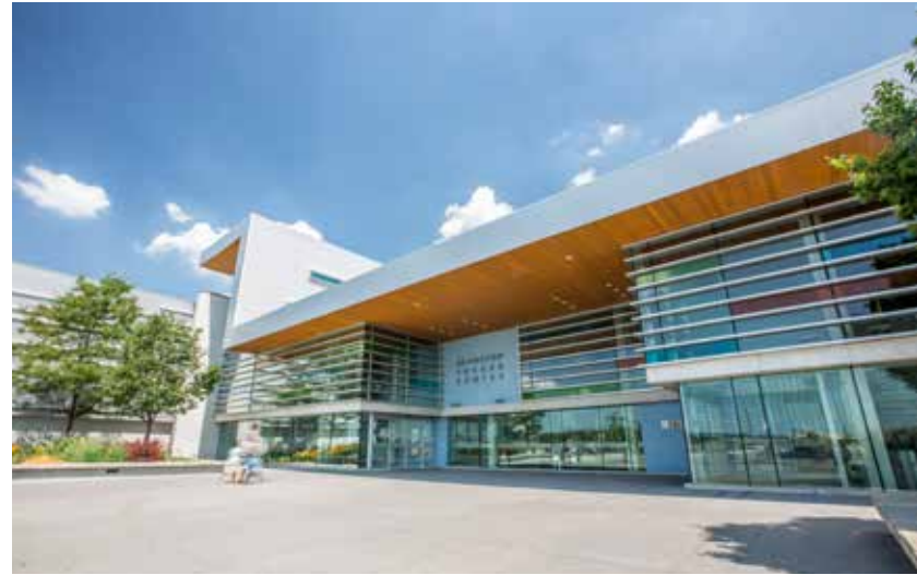
Fig 4.6.1 Brampton Soccer Centre Entrance
