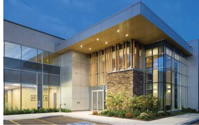
Fig 4.6.2 Building Entrance - Trailcon
