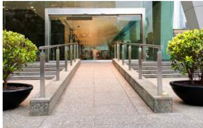
Fig 4.6.1 High Rise Accessible Entrance
