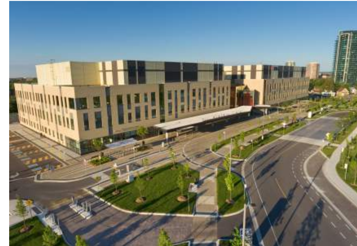
Fig 5.1.1 Peel Memorial Hospital
