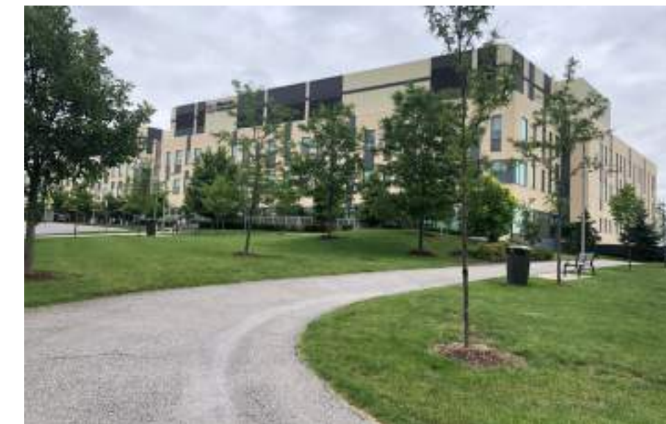
Fig 2.1.5 Peel Memorial Hospital
