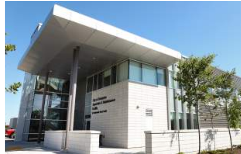
Fig 4.6.2 Brampton Apparatus and Maintenance Facility Entrance
