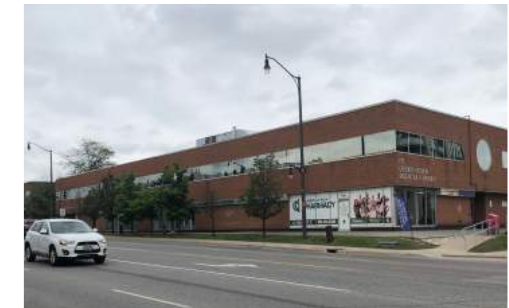
Fig 2.1.6 Office Building Along Centre Street
