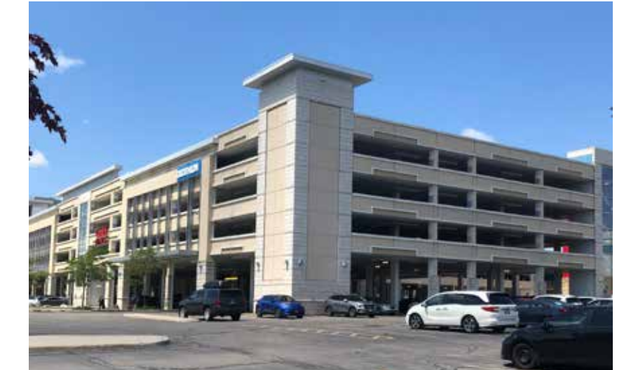
Fig 4.6.6 Aboveground Parking Garage, Bramalea City Centre
