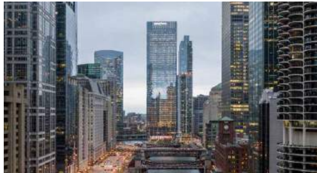
Fig 4.3.4 Salesforce Tower, Chicago, Goettsch Partners
