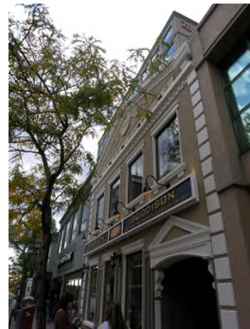
Building Façade Improvements
