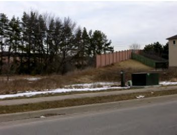
Residential Rail Noise Wall– Ravenscliffe Court
