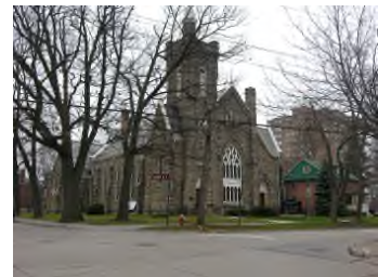
St Andrews Presbyterian - Church Street
