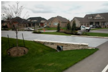
Springbrook Surface Run-off Treatment
