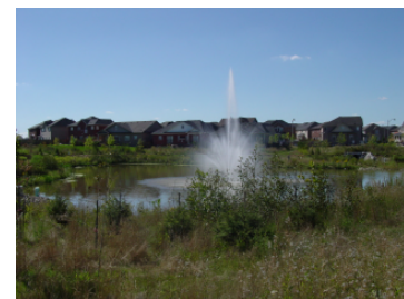
Danimar Stormwater Management Pond
