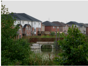
McClure Channel – Opportunity for Stormwater Recharge
