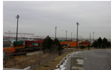
Brampton CN Intermodal Terminal
