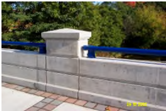
Main Street Bridge
