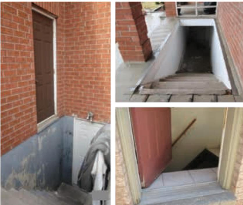
Examples of trip and fall hazards; unsafe and illegal access to secondary units.
