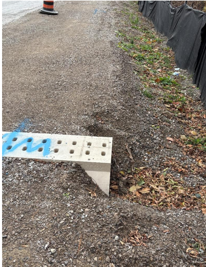
Figure 11 Wildlife culvert passage exposed, allowing wildlife to bypass and cross the road.
