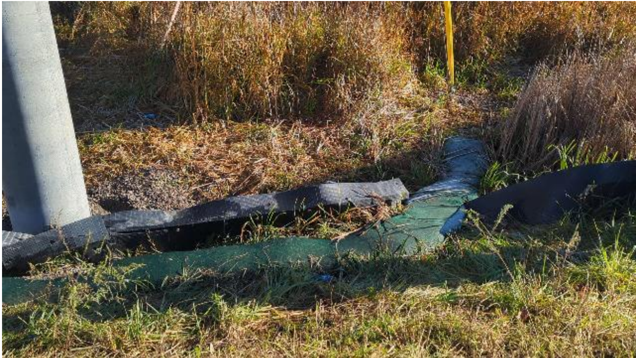
Figure 12 Improperly discarded silk sock causing damage to the exclusion fencing.
