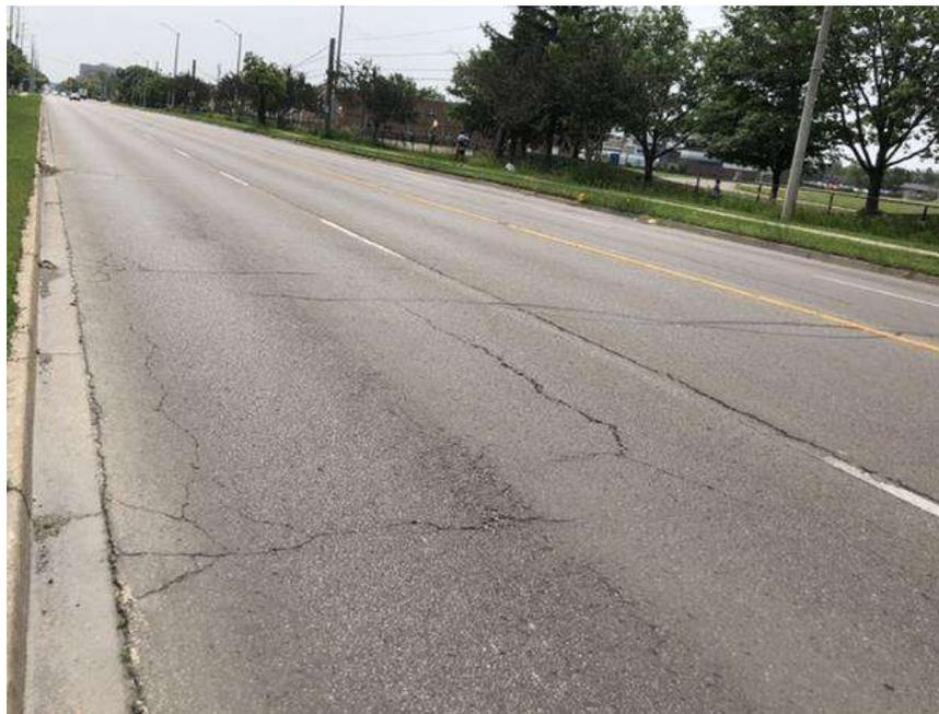
**Photograph 38 – Bramalea Road, Northbound, looking South, approximately 300 m South of Clark Boulevard, showing moderate to severe longitudinal and transverse cracking associated with moderate random cracking, slight to moderate pavement raveling and slight to moderate pavement edge cracking.**
