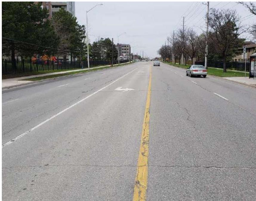
**Photograph 14 – Bramalea Road, looking North, near the intersection of Fleetwood Crescent and Bramalea Road, showing moderate longitudinal and transverse cracking associated with slight random cracking, slight pavement edge cracking and slight pavement raveling. Noting utility patching.**
