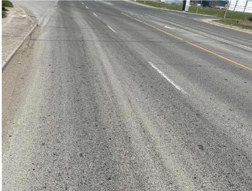
**Photograph 107 – Bramalea Road, Southbound, looking North, approximately 445 m South of Highway 407, showing slight longitudinal and transverse cracking associated with slight random cracking and slight to moderate pavement raveling.**
