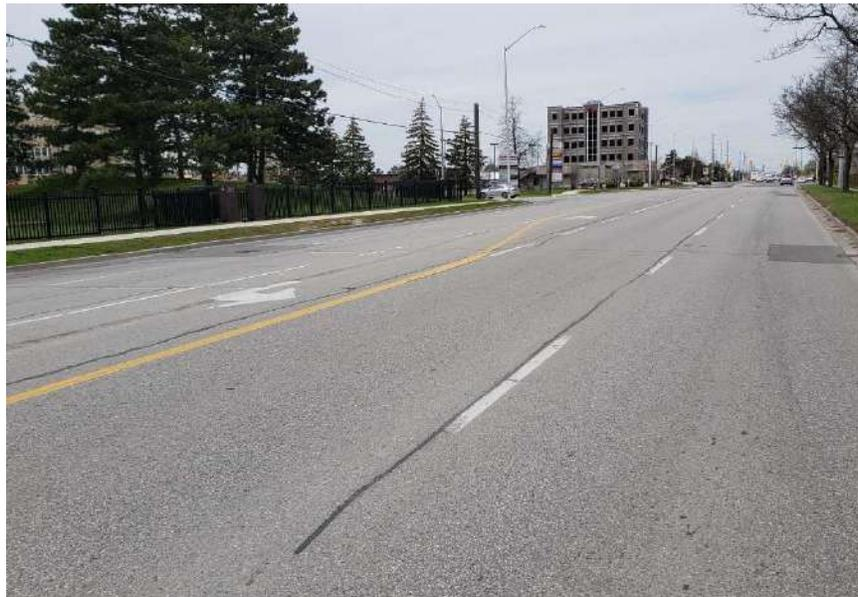
**Photograph 10 – Bramalea Road, Northbound, looking North, near the South intersection of Gates of Bramalea and Bramalea Road, showing moderate longitudinal and transverse cracking associated with slight random cracking, slight pavement edge cracking and slight pavement raveling. Noting sections of patching.**
