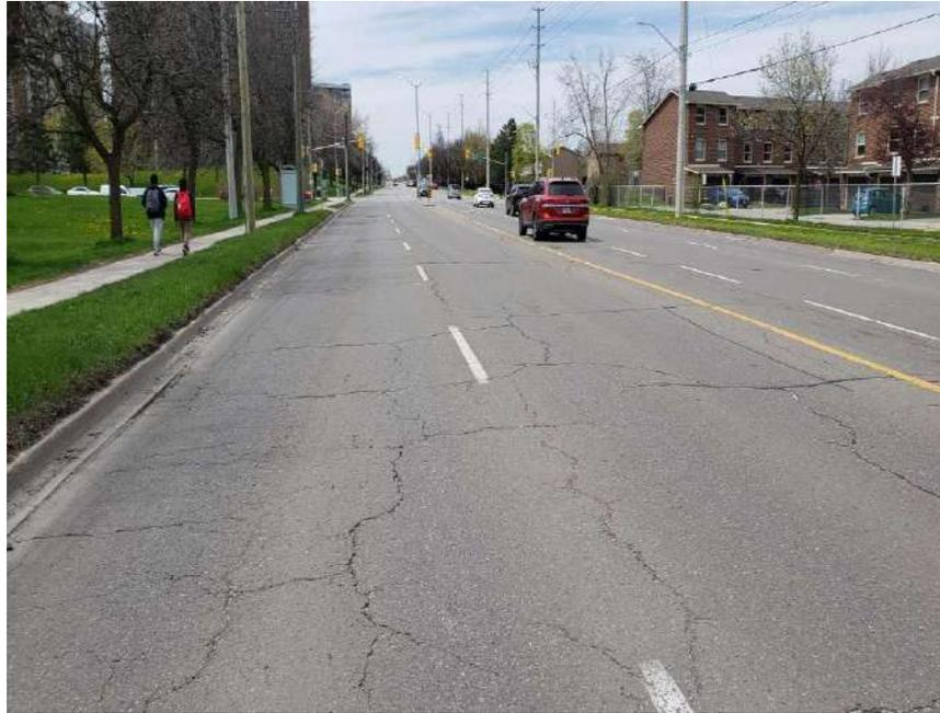
**Photograph 29 – Bramalea Road, Southbound, looking North, approximately 100 m South of Clark Boulevard, showing severe block cracking associated with moderate to severe longitudinal and transverse cracking, moderate random cracking, slight pavement raveling and slight to moderate pavement edge cracking.**
