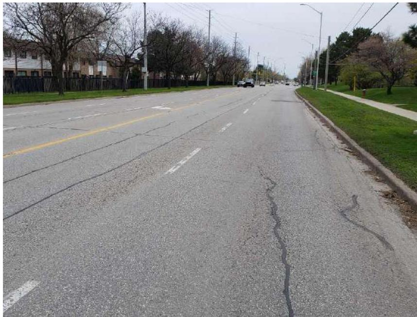
**Photograph 16 – Bramalea Road, Southbound, looking South, approximately 70 m South of Fleetwood Crescent, showing moderate to severe longitudinal and transverse cracking associated with slight to moderate random cracking, slight pavement depressions, slight to moderate pavement raveling and slight to moderate pavement edge cracking.**
