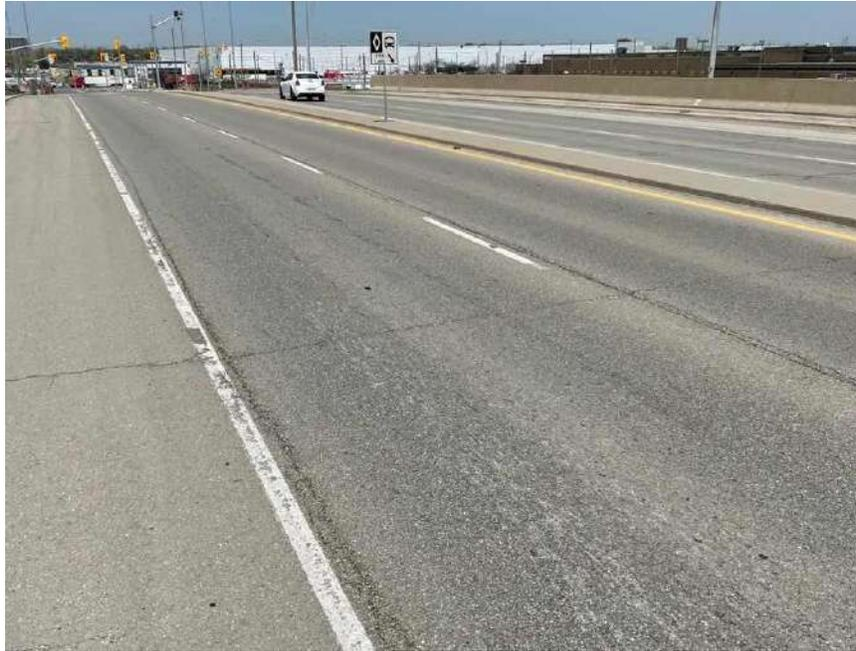
**Photograph 93 – Bramalea Road, Southbound, looking North, approximately 55 m South of Railway, showing moderate longitudinal and transverse cracking associated with slight random cracking and moderate pavement raveling.**
