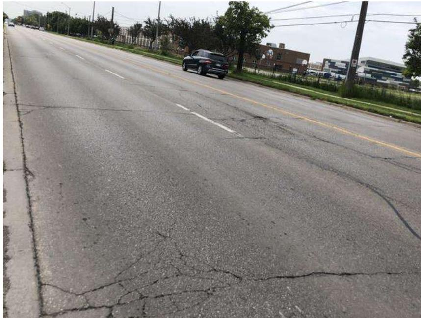
**Photograph 40 – Bramalea Road, Northbound, looking South, approximately 320 m North of Balmoral Drive, showing moderate to severe longitudinal and transverse cracking associated with moderate random cracking, moderate alligator cracking, slight potholes, slight to moderate pavement raveling and slight to moderate pavement edge cracking.**
