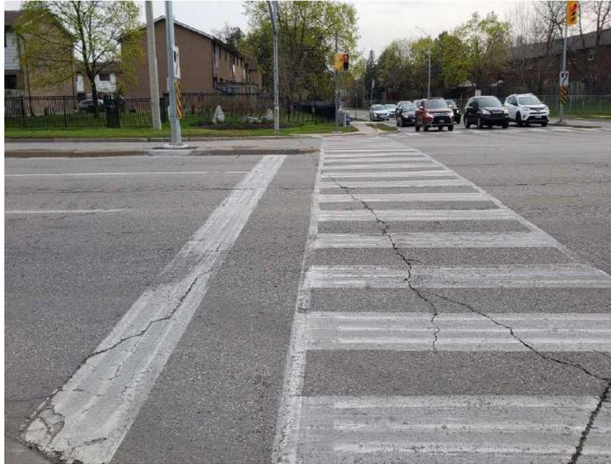
**Photograph 25 – Bramalea Road, Southbound, looking East, near the intersection of Bramalea Road and Clark Boulevard, showing moderate to severe longitudinal and transverse cracking associated with moderate to severe random cracking, slight to moderate pavement raveling and slight to moderate pavement edge cracking.**
