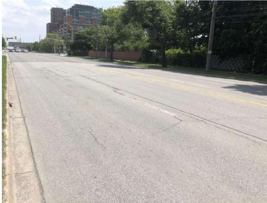
**Photograph 71 – Bramalea Road, Northbound, looking South, approximately 115 m North of Avondale Boulevard, showing moderate longitudinal and transverse cracking associated with slight random cracking, slight to moderate pavement raveling and slight pavement edge cracking.**
