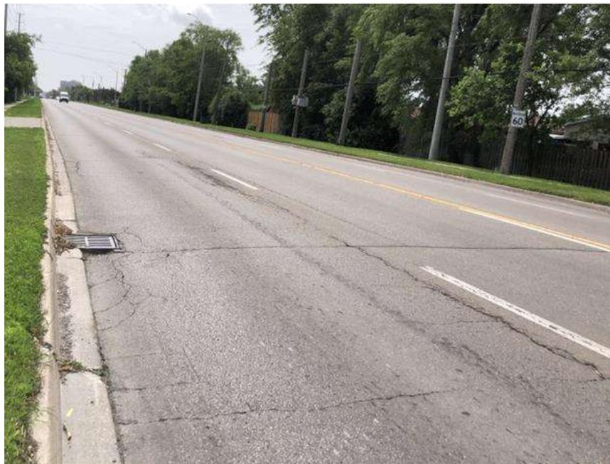
**Photograph 32 – Bramalea Road, Northbound, looking South, approximately 145 m South of Clark Boulevard, showing severe longitudinal and transverse cracking associated with slight to moderate random cracking, slight alligator cracking, slight to moderate pavement raveling, slight potholes and moderate pavement edge cracking.**
