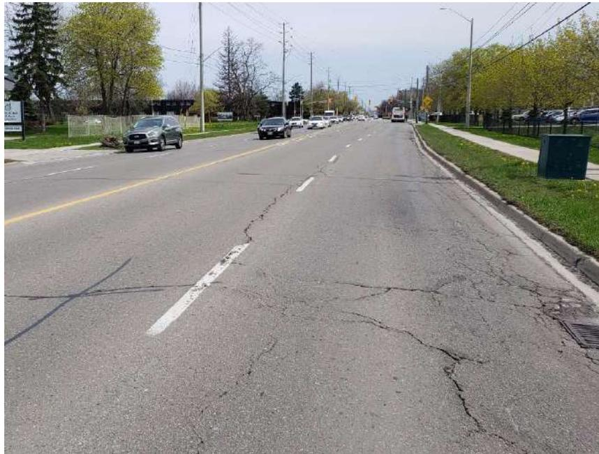
**Photograph 46 – Bramalea Road, Southbound, looking South, approximately 180 m North of Balmoral Drive, showing moderate to severe longitudinal and transverse cracking associated with moderate random cracking, moderate to severe alligator cracking, slight pavement raveling, slight pavement depressions, and moderate pavement edge cracking. Noting severe alligator cracking around catch basin.**
