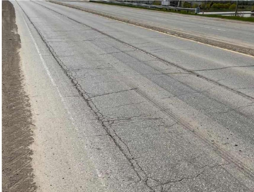
**Photograph 97 – Bramalea Road, Northbound, looking South, approximately 120 m North of the crossing over Highway 407, showing severe longitudinal and transverse cracking associated with severe random cracking, moderate alligator cracking, moderate block cracking and moderate pavement raveling.**
