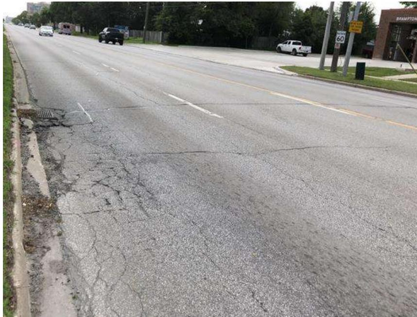
**Photograph 56 – Bramalea Road, Northbound, looking South, approximately 60 m North of Darras Court, showing moderate to severe longitudinal and transverse cracking associated with slight to moderate random cracking, moderate alligator cracking, slight to moderate pavement raveling, slight pavement depressions, and moderate pavement edge cracking. Noting severe alligator cracking around catch basin.**
