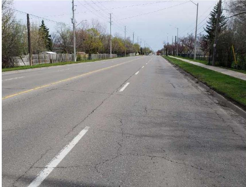
**Photograph 37 – Bramalea Road, Southbound, looking South, approximately 280 m South of Bramalea Road and Clark Boulevard, showing moderate to severe longitudinal and transverse cracking associated with moderate random cracking, slight to moderate block cracking, slight pavement raveling and slight to moderate pavement edge cracking.**
