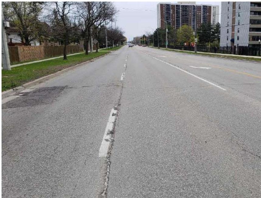
**Photograph 8 – Bramalea Road, Northbound, looking South, at the intersection of Kensington Road and Bramalea Road, showing moderate longitudinal and transverse cracking associated with moderate random cracking, slight pavement edge cracking and slight pavement raveling. Noting sections of patching.**
