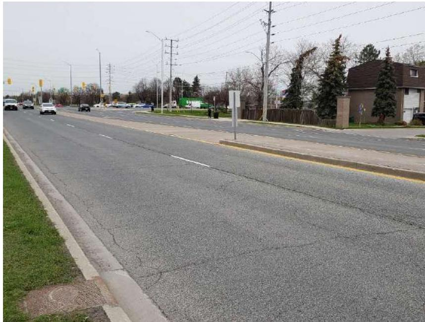
**Photograph 6 – Bramalea Road, Southbound, looking North, approximately 135 m South of Queen Street East, showing moderate longitudinal and transverse cracking associated with moderate random cracking, slight to moderate pavement edge cracking and slight pavement raveling.**
