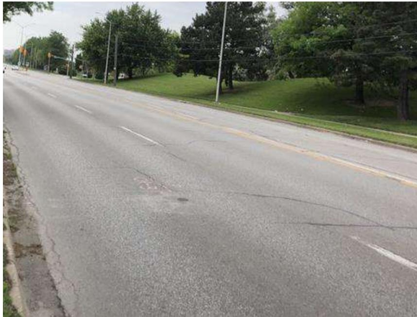
**Photograph 20 – Bramalea Road, Northbound, looking South, approximately 150 m South of Fleetwood Crescent, showing moderate longitudinal and transverse cracking associated with moderate random cracking, slight pavement depressions, slight to moderate pavement raveling, slight potholes and moderate to severe pavement edge cracking.**
