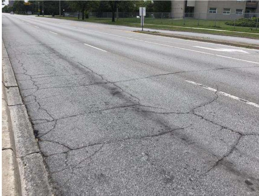
**Photograph 51 – Bramalea Road, Northbound, looking South, near the intersection of Bramalea Road and Balmoral Drive, showing moderate to severe longitudinal and transverse cracking associated with moderate random cracking, slight to moderate alligator cracking, moderate to severe block cracking, slight pavement raveling and moderate to severe pavement edge cracking.**
