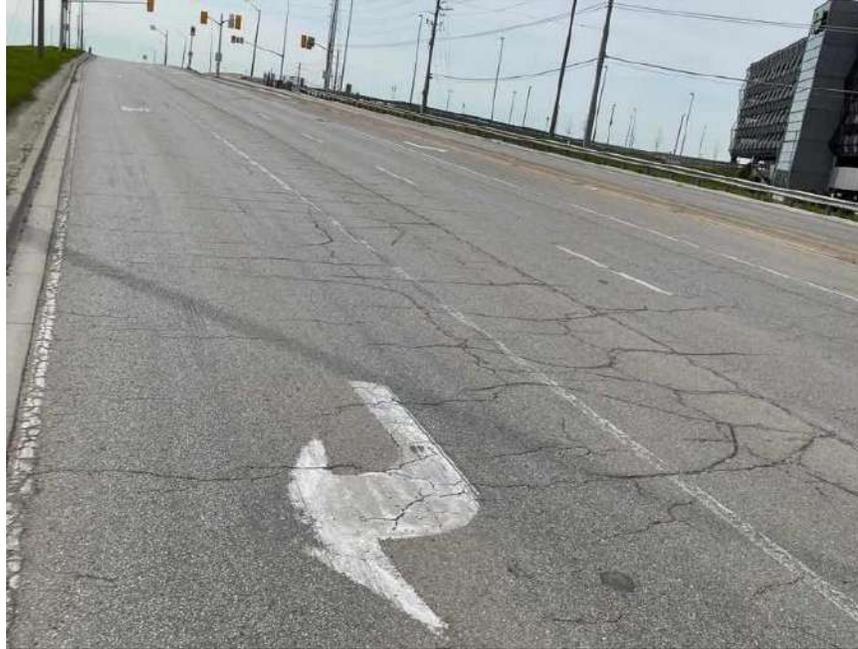
**Photograph 87 – Bramalea Road, Northbound, looking South, approximately 160 m South of Steeles Avenue East, showing severe longitudinal and transverse cracking associated with severe random cracking, severe block cracking, moderate alligator cracking, moderate pavement edge cracking and slight to moderate pavement raveling.**
