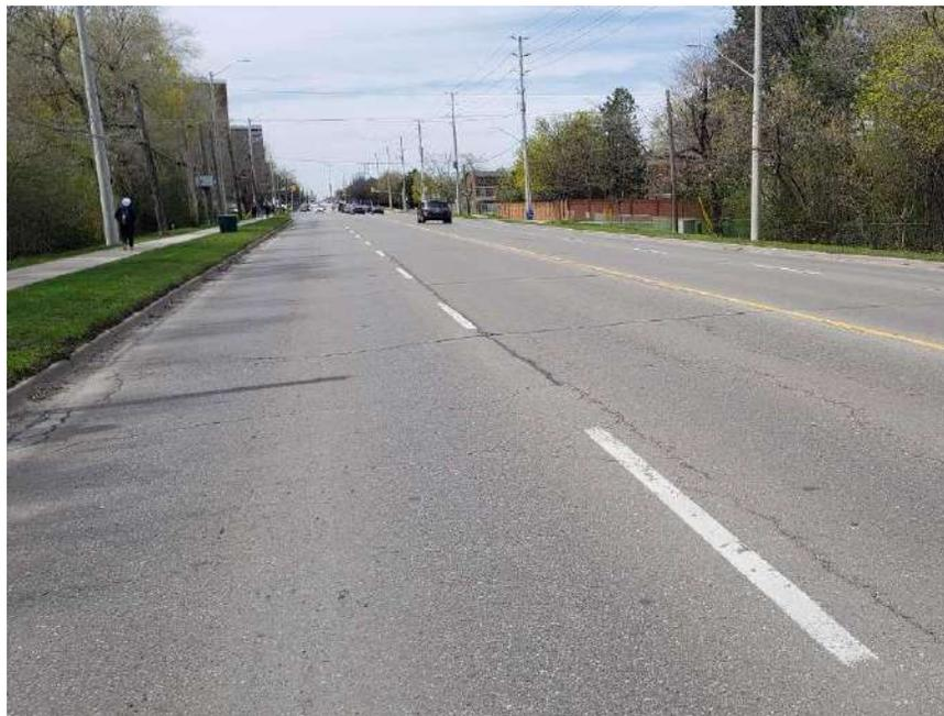
**Photograph 36 – Bramalea Road, Southbound, looking North, approximately 250 m South of Clark Boulevard, showing moderate longitudinal and transverse cracking associated with slight to moderate random cracking, slight pavement raveling and slight to moderate pavement edge cracking.**
