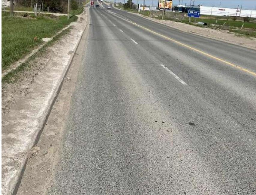
**Photograph 109 – Bramalea Road, Southbound, looking North, approximately 570 m South of Highway 407, showing slight to moderate longitudinal and transverse cracking associated with slight to moderate random cracking and slight to moderate pavement raveling.**
