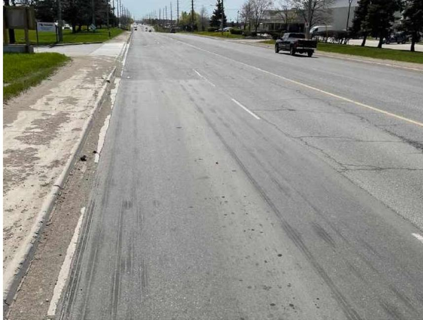
**Photograph 113 – Bramalea Road, Northbound, looking South, approximately 790 m South of Highway 407, showing severe longitudinal and transverse cracking associated with moderate to severe random cracking, severe block cracking, slight longitudinal construction joint and moderate pavement raveling. Noting sections of patching.**
