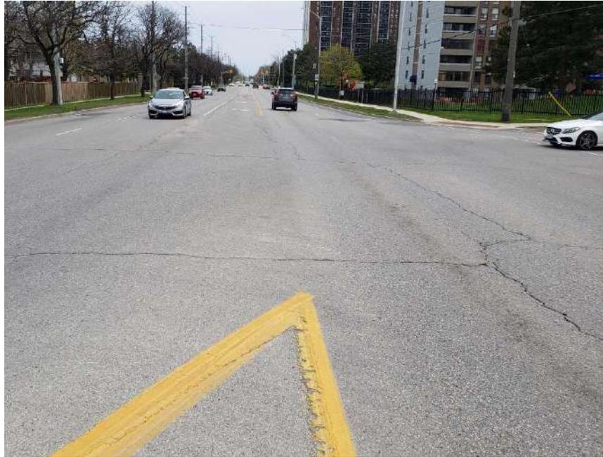
**Photograph 7 – Bramalea Road, looking South, near the intersection of Kensington Road and Bramalea Road, showing moderate to severe longitudinal and transverse cracking associated with slight to moderate random cracking and slight pavement raveling. Noting sections of patching.**
