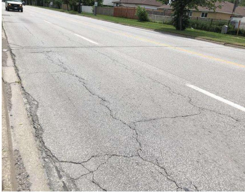
**Photograph 59 – Bramalea Road, Northbound, looking South, approximately 50 m South of Algonquin Boulevard, showing severe longitudinal and transverse cracking associated with moderate random cracking, moderate block cracking, slight pavement raveling and moderate to severe pavement edge cracking.**
