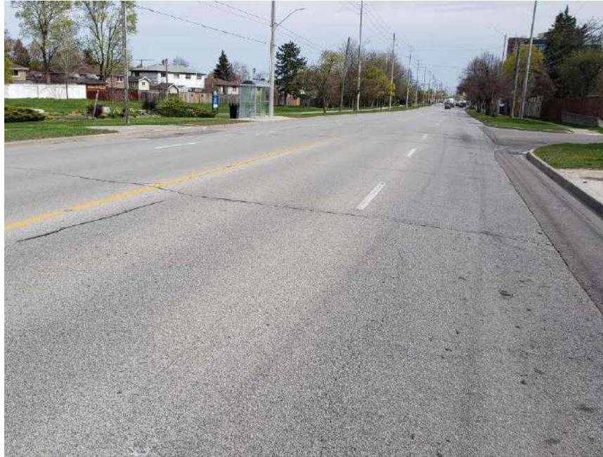
**Photograph 65 – Bramalea Road, Southbound, looking South, near the intersection of Bramalea Road and Alexandria Gate, showing moderate longitudinal and transverse cracking associated with slight random cracking and slight pavement raveling. Noting sections of patching along the pavement edge.**
