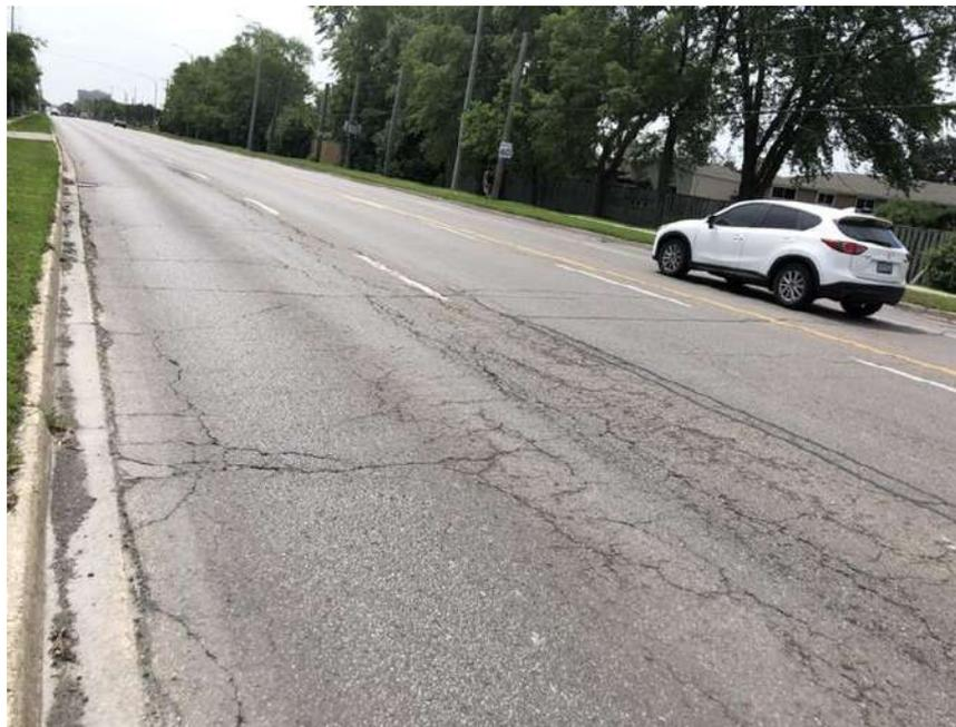
**Photograph 30 – Bramalea Road, Northbound, looking South, approximately 120 m South of Clark Boulevard, showing severe alligator cracking associated with moderate to severe longitudinal and transverse cracking, moderate to severe random cracking, moderate pavement raveling, moderate block cracking, slight pavement depressions and moderate to severe pavement edge cracking.**
