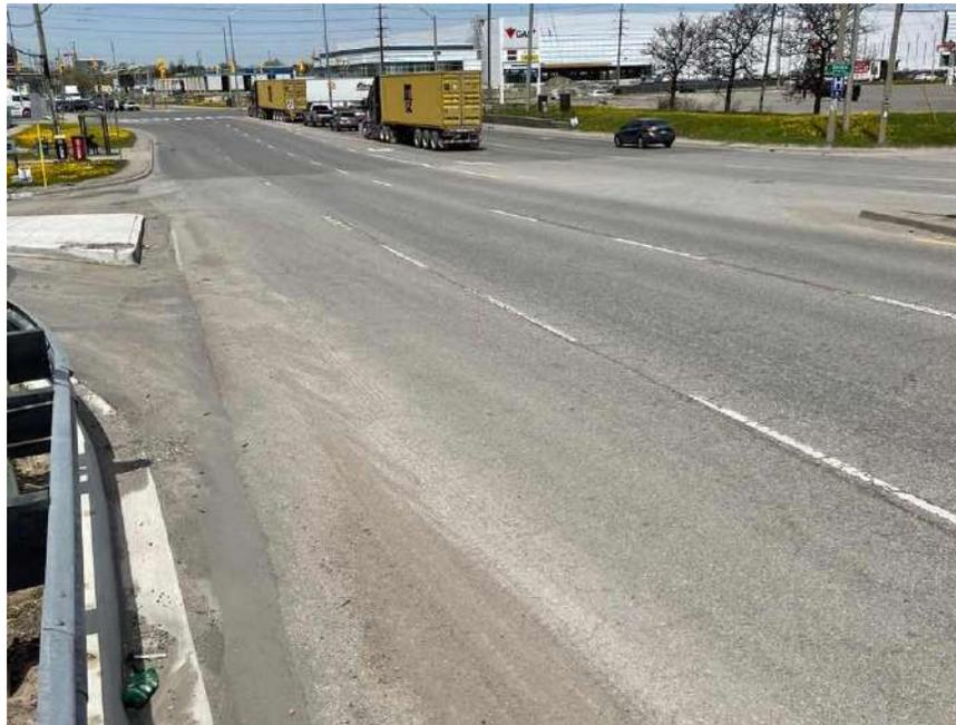
**Photograph 86 – Bramalea Road, Southbound, looking North, approximately 140 m South of Steeles Avenue East, showing moderate longitudinal and transverse cracking associated with slight to moderate random cracking, slight block cracking and slight to moderate pavement raveling.**
