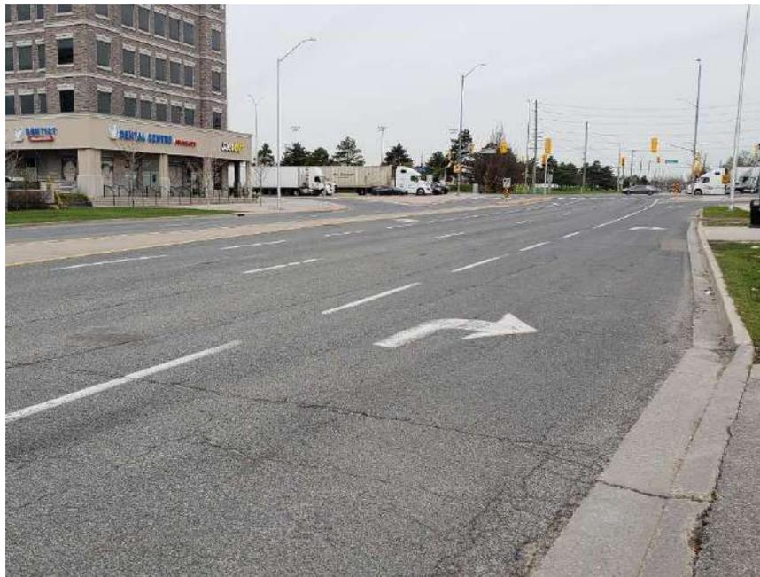
**Photograph 4 – Bramalea Road, Northbound, looking North, approximately 105 m South of Queen Street East, showing moderate longitudinal and transverse cracking associated with slight to moderate random cracking, slight block cracking, slight to moderate alligator cracking, slight potholes, moderate to severe pavement edge cracking and slight pavement raveling. Noting sections of patching.**
