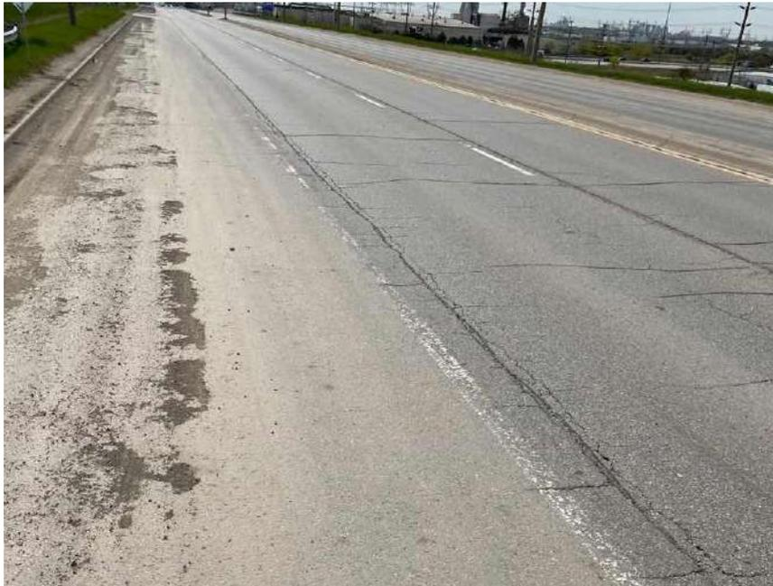
**Photograph 94 – Bramalea Road, Northbound, looking South, approximately 100 m South of Railway, showing severe longitudinal and transverse cracking associated with moderate random cracking, moderate block cracking, moderate pavement raveling and moderate pavement edge cracking.**
