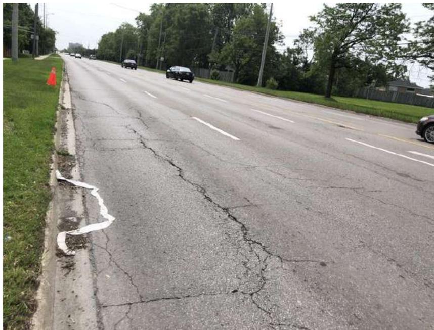
**Photograph 28 – Bramalea Road, Northbound, looking South, approximately 90 m South of Clark Boulevard, showing moderate to severe longitudinal and transverse cracking associated with moderate to severe random cracking, slight to moderate alligator cracking, slight to moderate pavement raveling and moderate pavement edge cracking.**
