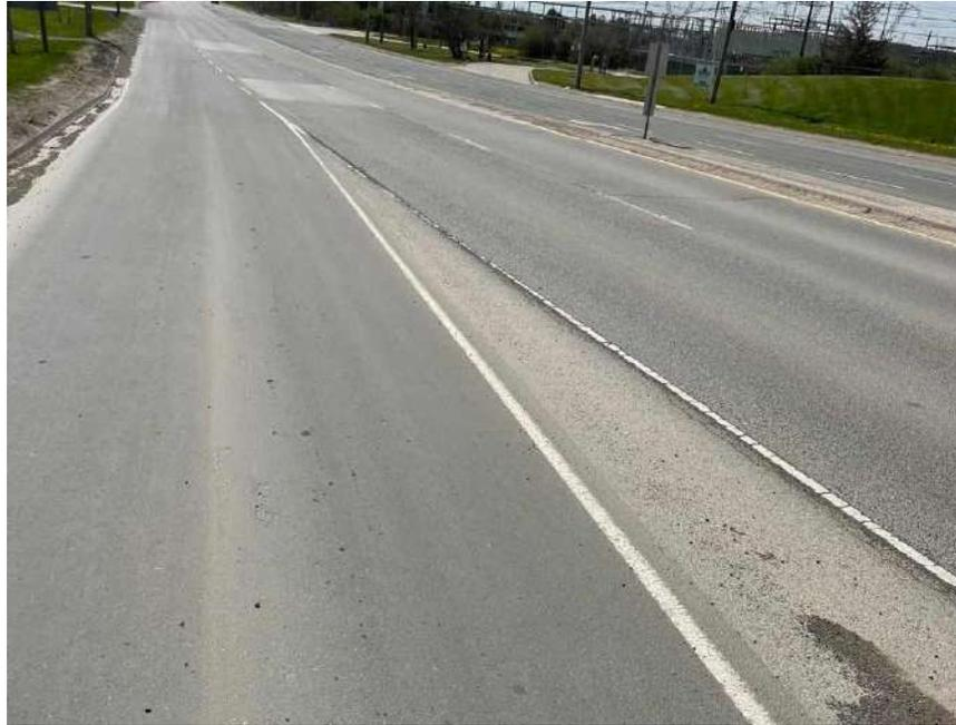
**Photograph 103 – Bramalea Road, Northbound, looking South, approximately 290 m South of Highway 407, showing slight to moderate longitudinal and transverse cracking associated with slight random cracking, slight alligator cracking and slight pavement raveling.**
