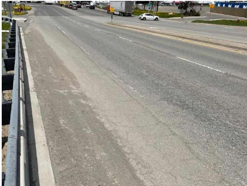
**Photograph 88 – Bramalea Road, Southbound, looking North, approximately 170 m South of Steeles Avenue East, showing moderate to severe longitudinal and transverse cracking associated with severe random cracking, severe block cracking, moderate alligator cracking, moderate pavement edge cracking and moderate pavement raveling.**
