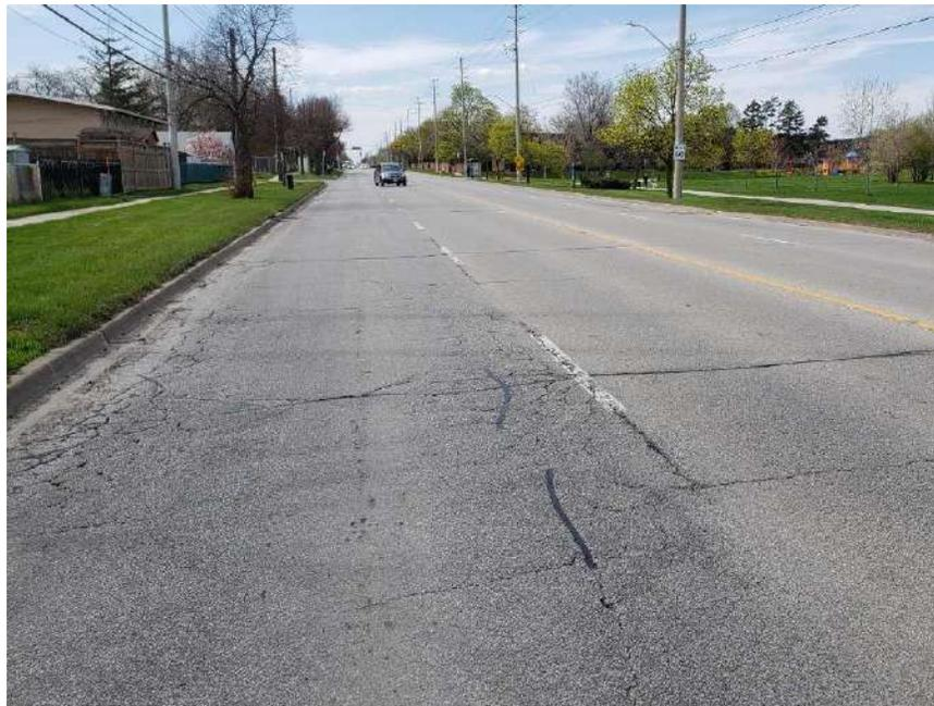
**Photograph 60 – Bramalea Road, Southbound, looking North, approximately 75 m South of Algonquin Boulevard, showing moderate to severe longitudinal and transverse cracking associated with moderate random cracking, slight pavement depressions, moderate pavement raveling, severe alligator cracking and moderate to severe pavement edge cracking.**
