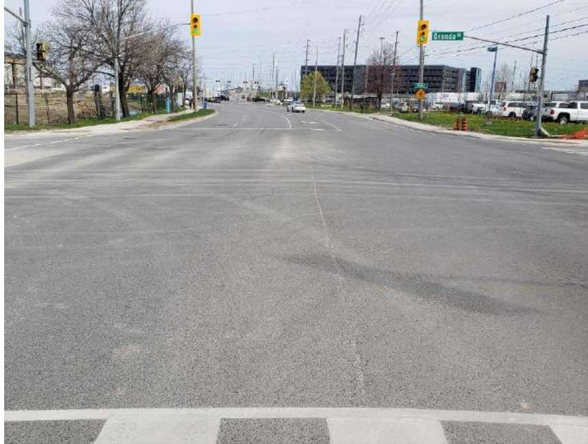
**Photograph 81 – Bramalea Road, looking South, near the intersection of Bramalea Road and Oronda Road, showing slight to moderate longitudinal and transverse cracking associated with slight random cracking and slight pavement raveling.**
