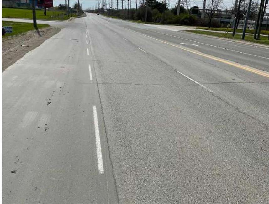
**Photograph 105 – Bramalea Road, Northbound, looking South, approximately 370 m South of Highway 407, showing moderate longitudinal and transverse cracking associated with slight random cracking, slight longitudinal construction joint and slight to moderate pavement raveling.**
