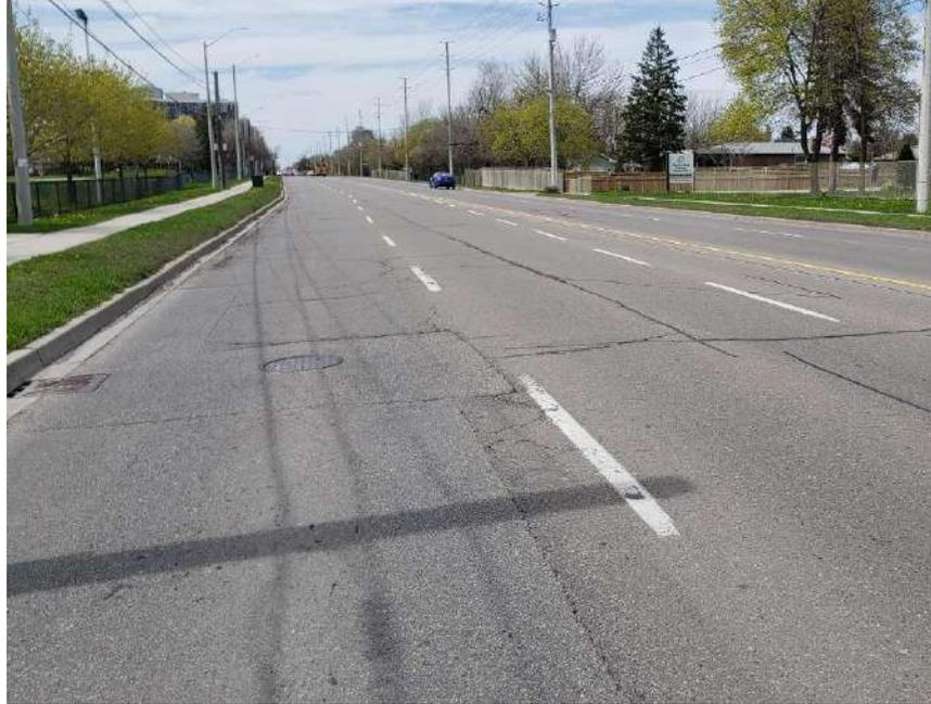
**Photograph 47 – Bramalea Road, Southbound, looking North, approximately 100 m North of Balmoral Drive, showing moderate to severe longitudinal and transverse cracking associated with moderate random cracking, slight alligator cracking, slight pavement raveling and moderate to severe pavement edge cracking. Noting sections of patching.**
