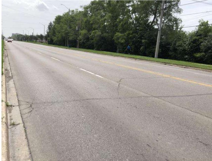
**Photograph 35 – Bramalea Road, Northbound, looking South, approximately 200 m South of Clark Boulevard, showing moderate longitudinal and transverse cracking associated with slight to moderate random cracking, slight alligator cracking, slight pavement raveling and slight to moderate pavement edge cracking.**
