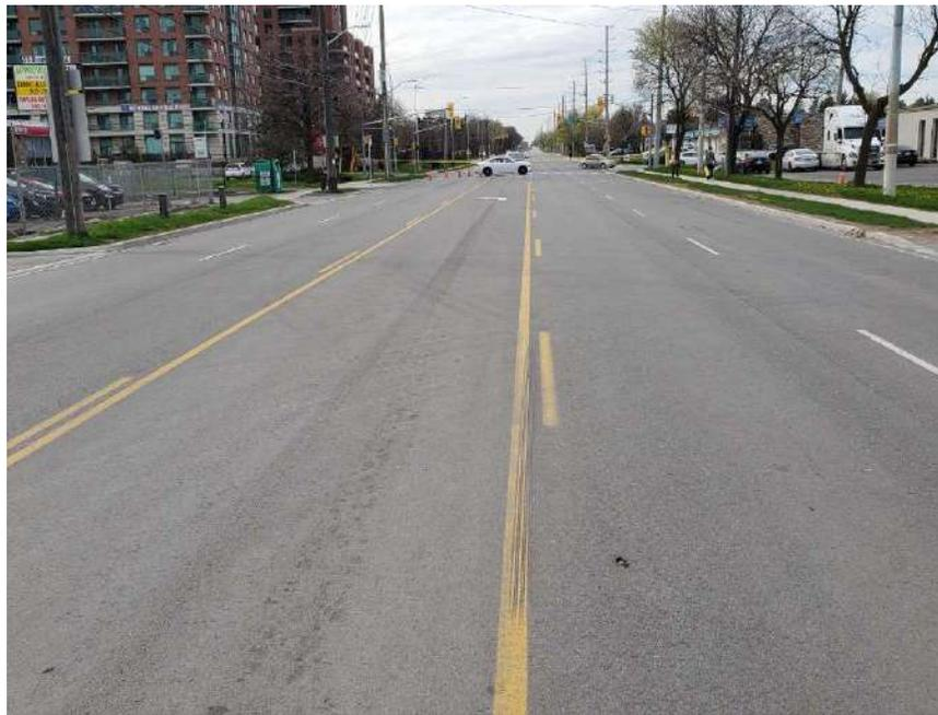
**Photograph 78 – Bramalea Road, looking North, approximately 90 m South of Bramalea Road/East Drive, showing relatively newly paved asphalt concrete.**
