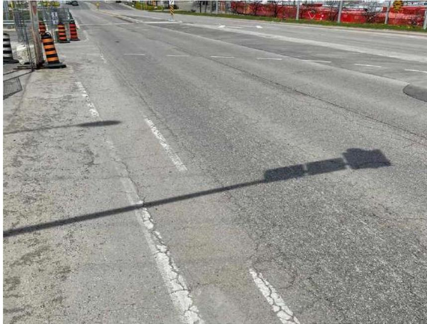
**Photograph 91 – Bramalea Road, Southbound, looking North, approximately 100 m North of Railway, showing moderate to severe longitudinal and transverse cracking associated with moderate random cracking, moderate to severe block cracking, moderate alligator cracking and moderate pavement raveling.**
