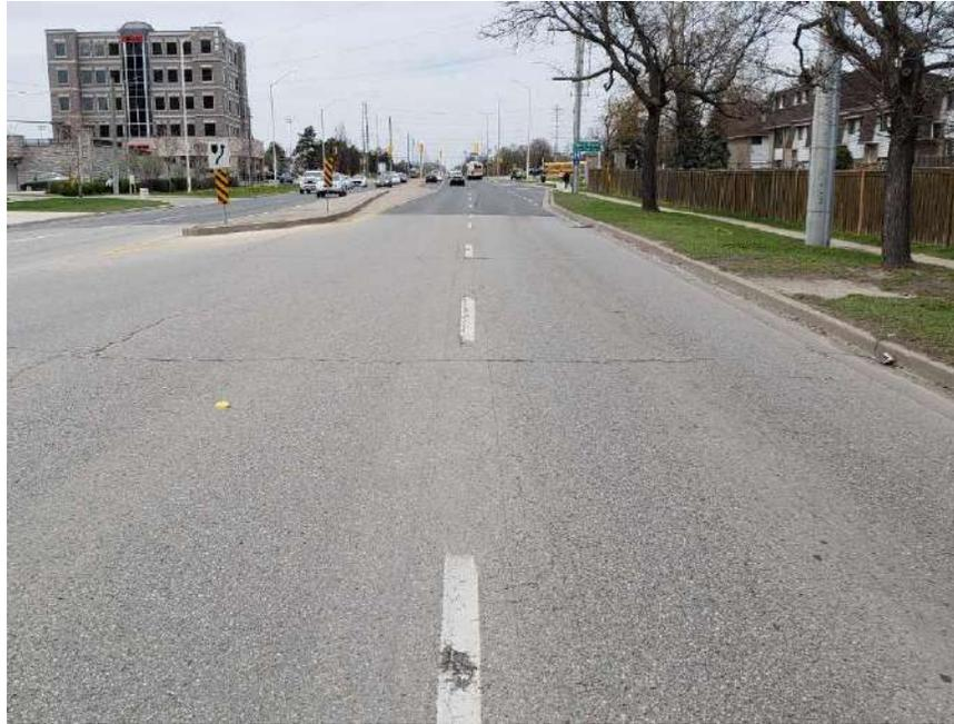
**Photograph 9 – Bramalea Road, Northbound, looking North, near the intersection of Kensington Road and Bramalea Road, showing moderate longitudinal and transverse cracking associated with slight random cracking, slight pavement edge cracking and slight pavement raveling.**
