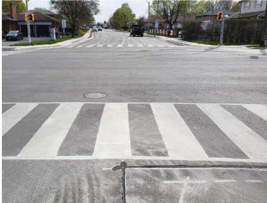
**Photograph 73 – Bramalea Road, looking West, near the intersection of Bramalea Road and Avondale Boulevard, showing slight longitudinal and transverse cracking associated with slight random cracking. Noting sections of patching.**
