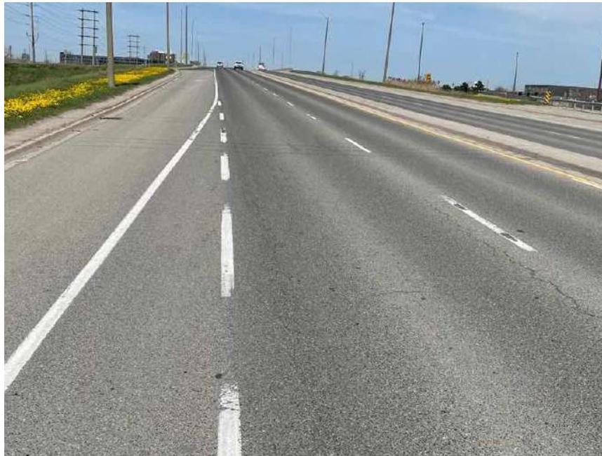
**Photograph 102 – Bramalea Road, Southbound, looking North, approximately 235 m South of Highway 407, showing slight to moderate longitudinal and transverse cracking associated with slight to moderate random cracking and slight to moderate pavement raveling.**
