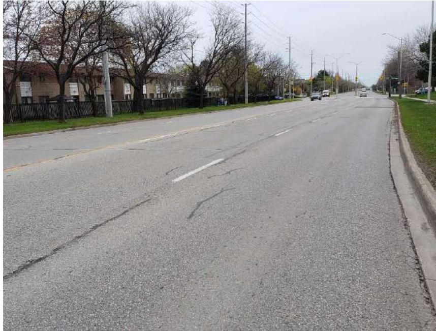
**Photograph 19 – Bramalea Road, Southbound, looking South, approximately 150 m South of Fleetwood Crescent, showing moderate to severe longitudinal and transverse cracking associated with moderate random cracking, slight pavement depressions, slight to moderate pavement raveling and slight pavement edge cracking.**
