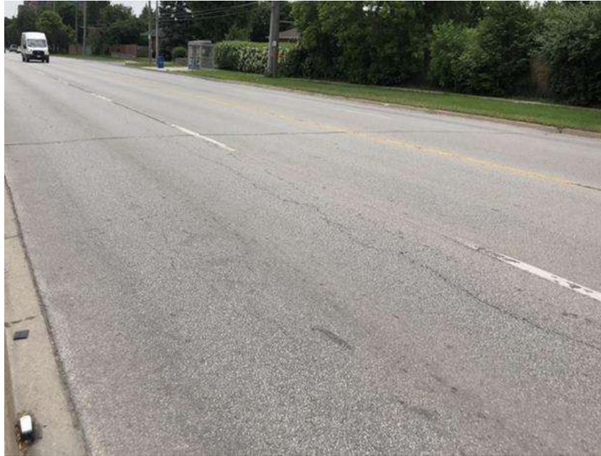
**Photograph 63 – Bramalea Road, Northbound, looking South, approximately 75 m North of Alexandria Gate, showing moderate longitudinal and transverse cracking associated with slight random cracking, slight alligator cracking, slight pavement raveling and slight pavement edge cracking.**
