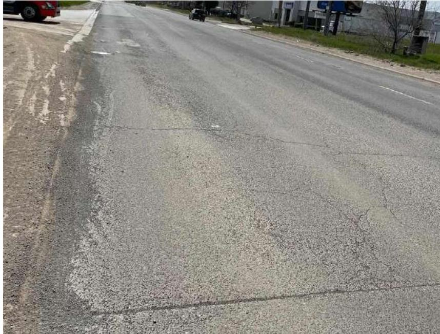
**Photograph 111 – Bramalea Road, Northbound, looking South, approximately 700 m South of Highway 407, showing moderate longitudinal and transverse cracking associated with moderate random cracking, slight block cracking and moderate to severe pavement raveling.**
