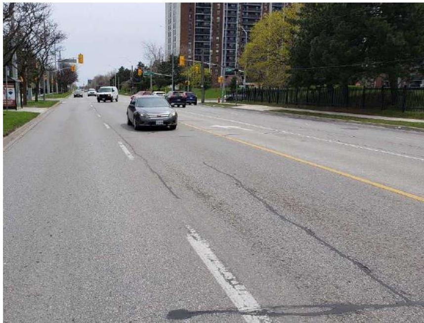
**Photograph 12 – Bramalea Road, Northbound, looking South, approximately 70 m North of Fleetwood Crescent, showing slight to moderate longitudinal and transverse cracking associated with slight random cracking, slight pavement edge cracking and slight to moderate pavement raveling.**
