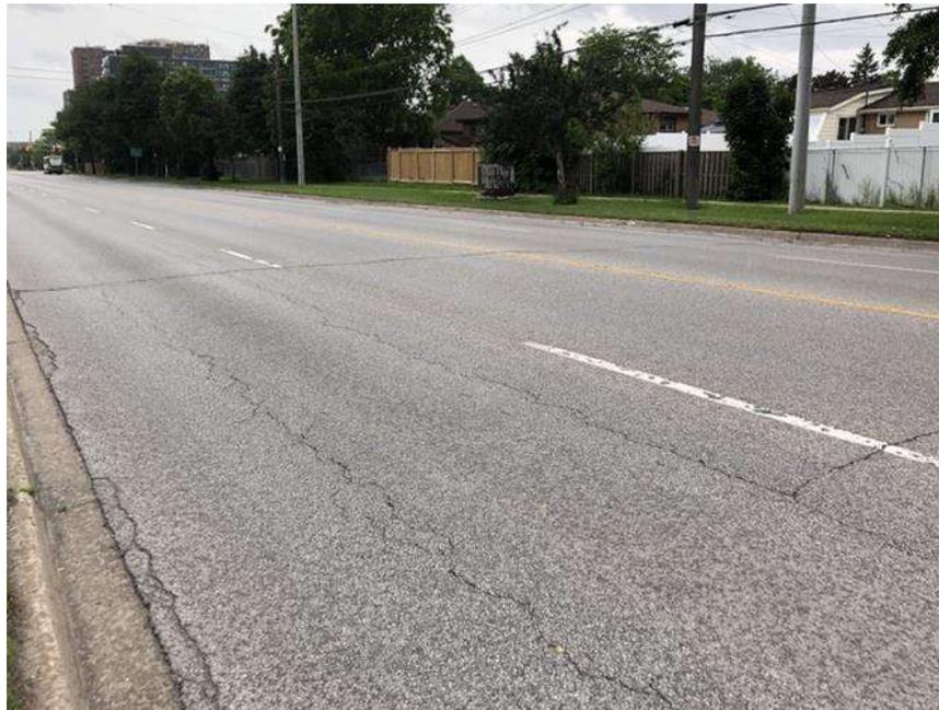
**Photograph 68 – Bramalea Road, Northbound, looking South, approximately 100 m South of Alexandria Gate, showing moderate longitudinal and transverse cracking associated with slight random cracking, moderate pavement raveling, slight alligator cracking, slight to moderate block cracking and moderate pavement edge cracking.**
