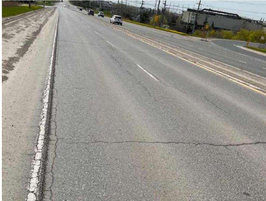
**Photograph 99 – Bramalea Road, Northbound, looking South, approximately 90 m South of Highway 407, showing moderate to severe longitudinal and transverse cracking associated with moderate to severe random cracking, moderate alligator cracking, severe pavement edge cracking and moderate pavement raveling.**
