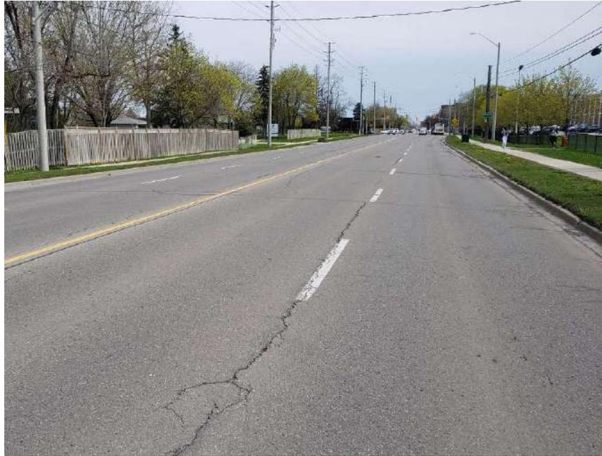
**Photograph 43 – Bramalea Road, Southbound, looking South, approximately 210 m North of Balmoral Drive, showing moderate to severe longitudinal and transverse cracking associated with slight to moderate random cracking, slight pavement raveling and slight to moderate pavement edge cracking.**
