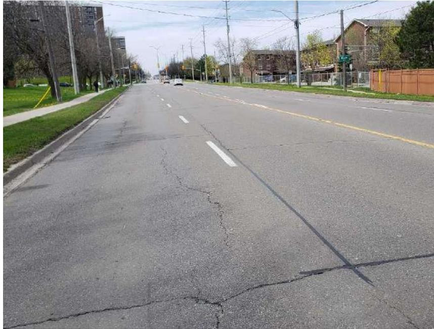
**Photograph 33 – Bramalea Road, Southbound, looking North, approximately 170 m South of Clark Boulevard, showing moderate to severe longitudinal and transverse cracking associated with slight to moderate random cracking, slight pavement raveling and slight to moderate pavement edge cracking.**
