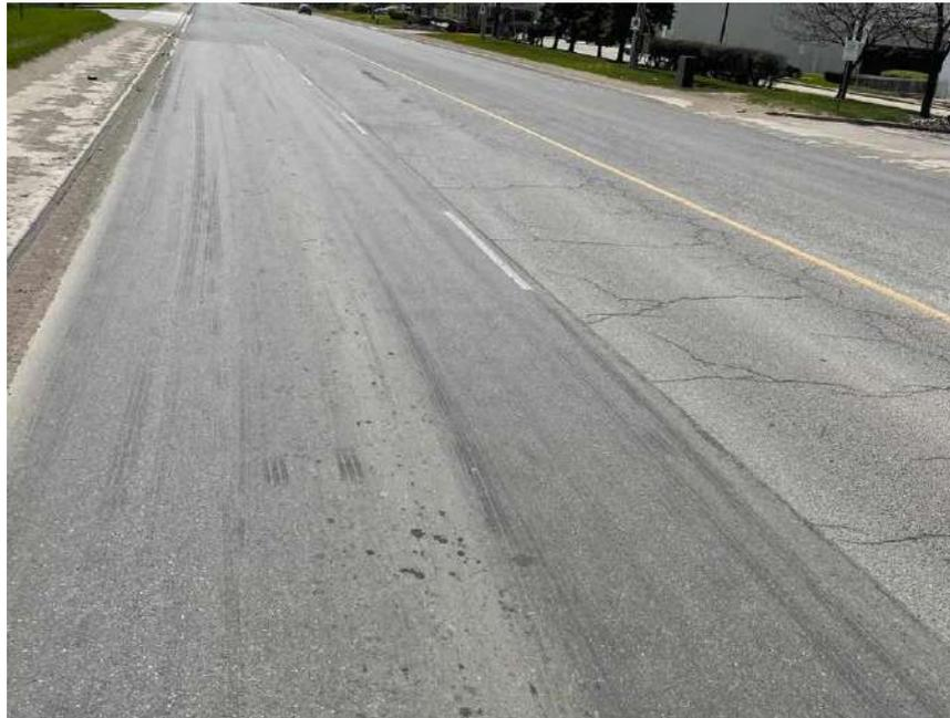
**Photograph 112 – Bramalea Road, Northbound, looking South, approximately 720 m South of Highway 407, showing severe longitudinal and transverse cracking associated with moderate to severe random cracking, severe blocking cracking, slight longitudinal construction joint and moderate pavement raveling. Noting sections of patching.**
