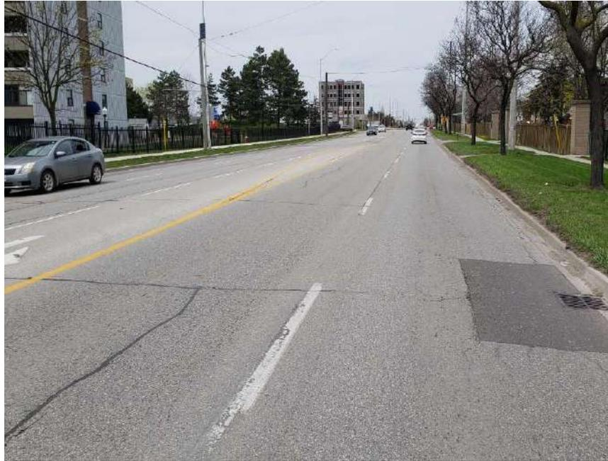
**Photograph 13 – Bramalea Road, Northbound, looking North, approximately 85 m North of Fleetwood Crescent, showing moderate longitudinal and transverse cracking associated with slight random cracking, slight to moderate pavement edge cracking and slight to moderate pavement raveling. Noting patching around catch basin.**
