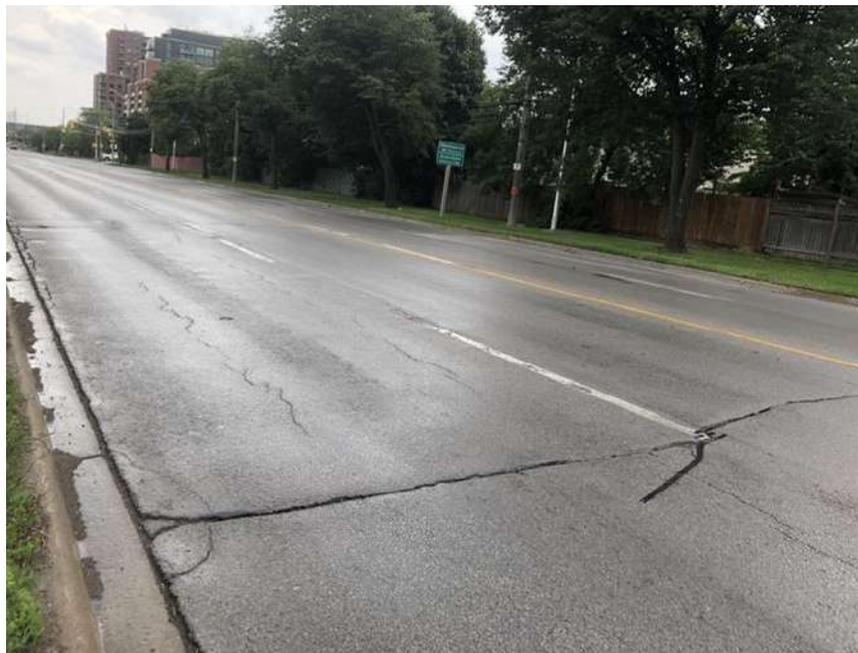
**Photograph 70 – Bramalea Road, Northbound, looking South, approximately 155 m North of Avondale Boulevard, showing moderate to severe longitudinal and transverse cracking associated with slight to moderate random cracking, slight pavement raveling and slight to moderate pavement edge cracking.**
