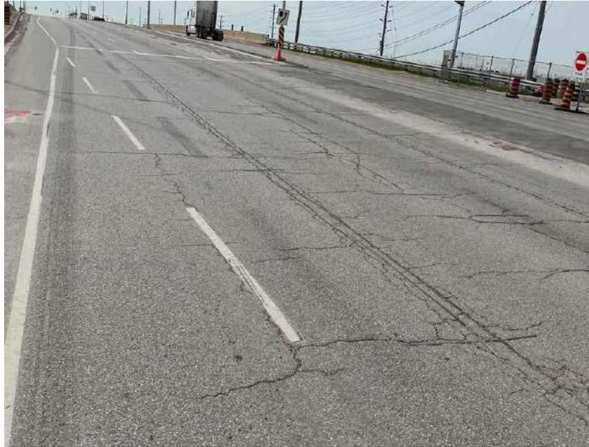
**Photograph 89 – Bramalea Road, Northbound, looking South, approximately 150 m North of Railway, showing severe longitudinal and transverse cracking associated with severe random cracking, severe block cracking, moderate alligator cracking and moderate pavement raveling.**
