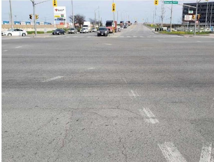
**Photograph 83 – Bramalea Road, Southbound, looking South, near the intersection of Bramalea Road and Steeles Avenue East, showing moderate longitudinal and transverse cracking associated with moderate random cracking, slight block cracking and slight pavement raveling.**
