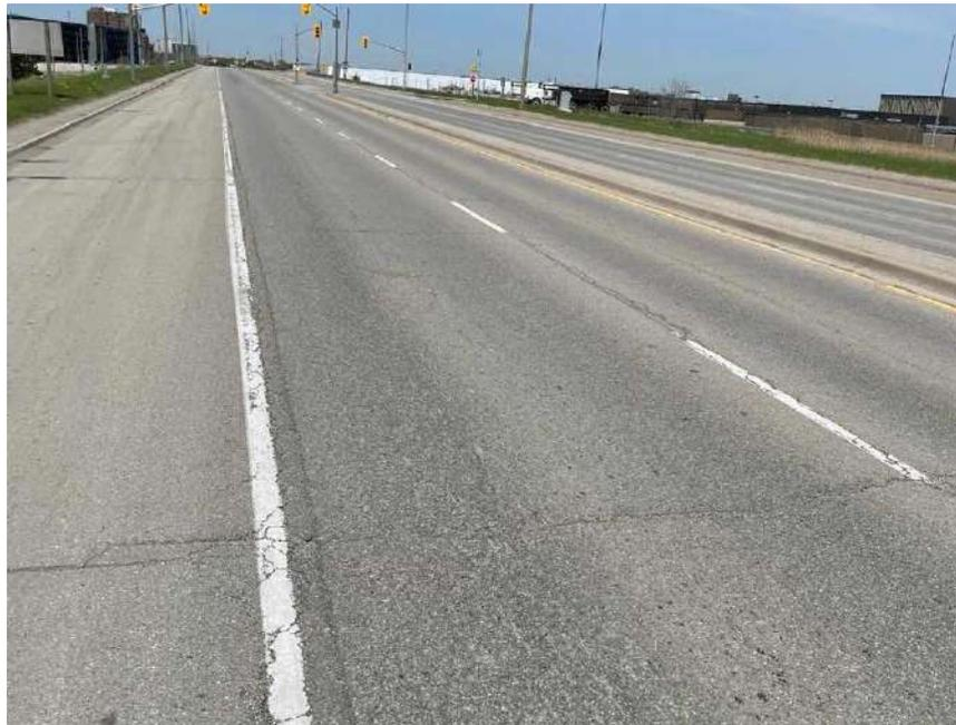
**Photograph 98 – Bramalea Road, Southbound, looking North, approximately 80 m North of the crossing over Highway 407, showing moderate longitudinal and transverse cracking associated with moderate random cracking, moderate pavement raveling and slight alligator cracking.**
