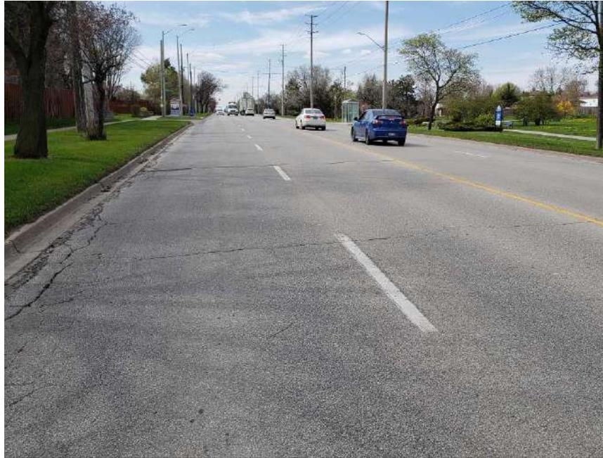
**Photograph 67 – Bramalea Road, Southbound, looking North, approximately 60 m South of Alexandria Gate, showing moderate longitudinal and transverse cracking associated with slight random cracking, slight to moderate pavement raveling and severe pavement edge cracking.**
