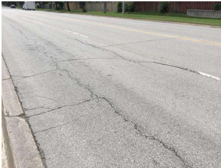
**Photograph 66 – Bramalea Road, Northbound, looking South, near the intersection of Bramalea Road and Alexandria Gate, showing severe longitudinal and transverse cracking associated with moderate random cracking, moderate block cracking, slight alligator cracking, and slight pavement raveling.**
