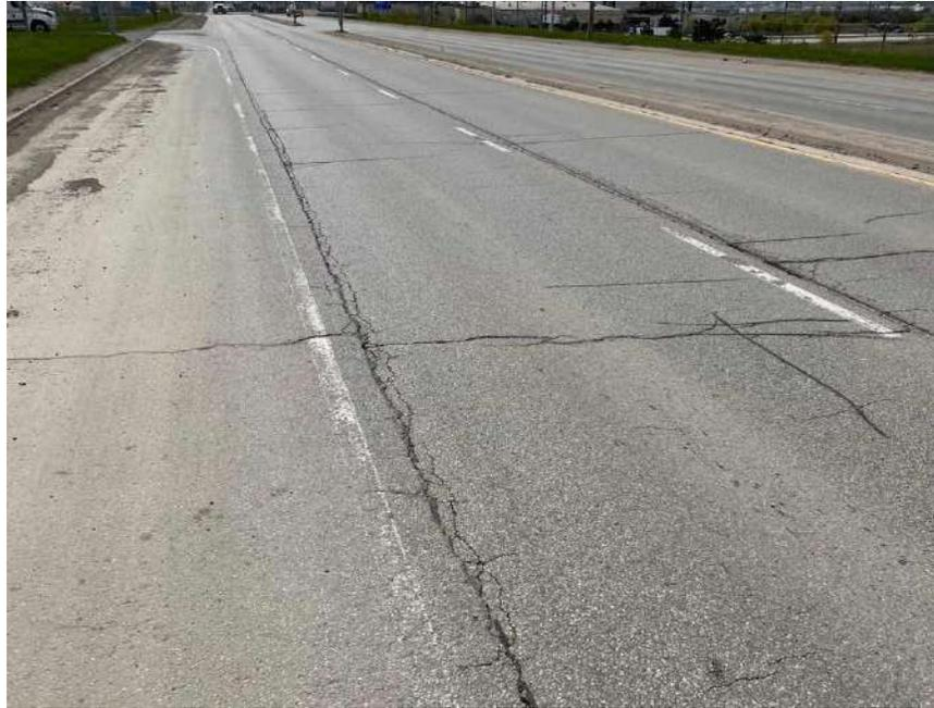
**Photograph 95 – Bramalea Road, Northbound, looking South, approximately 130 m South of Railway, showing severe longitudinal and transverse cracking associated with moderate random cracking, moderate pavement raveling and slight block cracking.**
