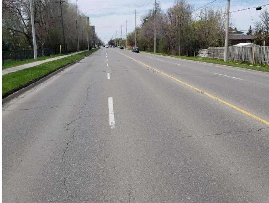
**Photograph 39 – Bramalea Road, Southbound, looking North, approximately 325 m South of Clark Boulevard, showing moderate to severe longitudinal and transverse cracking associated with slight to moderate random cracking, slight pavement raveling and slight to moderate pavement edge cracking.**
