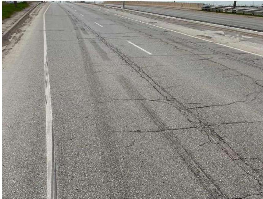
**Photograph 90 – Bramalea Road, Northbound, looking South, approximately 100 m North of Railway, showing severe longitudinal and transverse cracking associated with severe random cracking, severe block cracking, moderate alligator cracking and moderate pavement raveling.**
