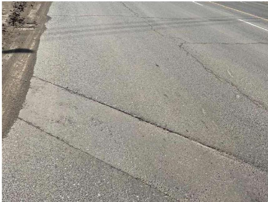
**Photograph 108 – Bramalea Road, Northbound, looking South, approximately 515 m South of Highway 407, showing moderate longitudinal and transverse cracking associated with moderate random cracking and slight to moderate pavement raveling. Noting utility patching.**
