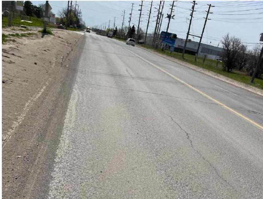
**Photograph 110 – Bramalea Road, Northbound, looking South, approximately 645 m South of Highway 407, showing moderate longitudinal and transverse cracking associated with slight to moderate random cracking and moderate pavement raveling.**
