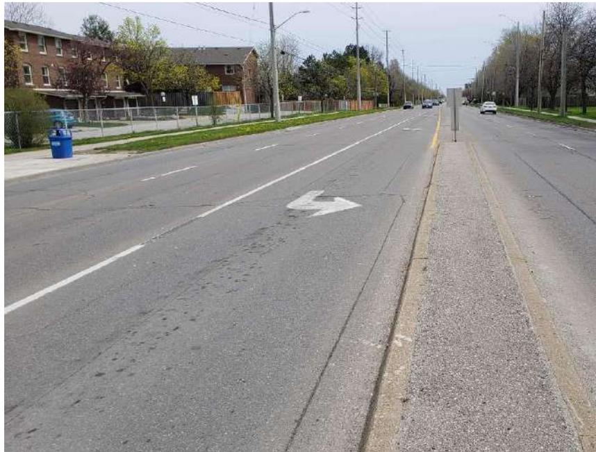
**Photograph 26 – Bramalea Road, Northbound, looking South, near the intersection of Bramalea Road and Clark Boulevard, showing moderate longitudinal and transverse cracking associated with slight to moderate random cracking, slight pavement raveling and slight pavement edge cracking.**
