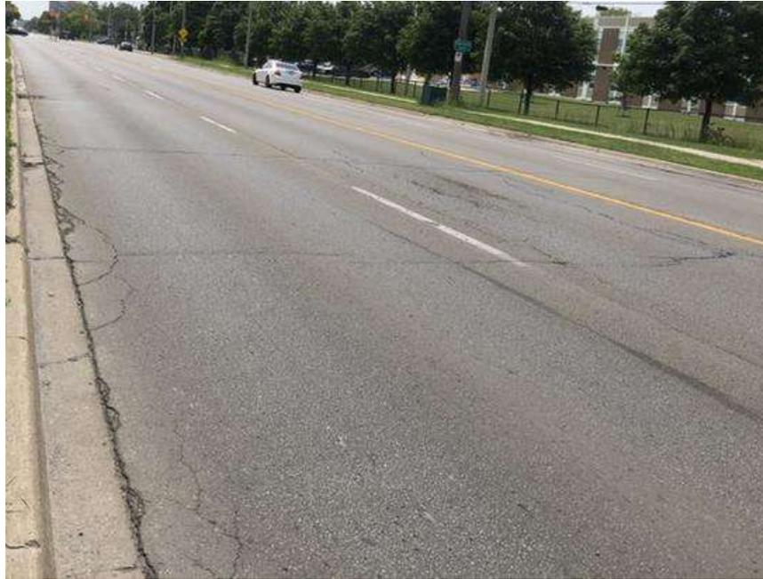
**Photograph 45 – Bramalea Road, Northbound, looking South, approximately 200 m North of Balmoral Drive, showing moderate to severe longitudinal and transverse cracking associated with slight to moderate random cracking, slight pavement depressions, slight to moderate pavement raveling and moderate to severe pavement edge cracking.**
