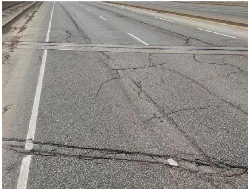
**Photograph 92 – Bramalea Road, Northbound, looking South, near Railway, showing severe longitudinal and transverse cracking associated with severe random cracking, moderate block cracking, moderate alligator cracking, moderate pavement raveling and slight pavement edge cracking.**
