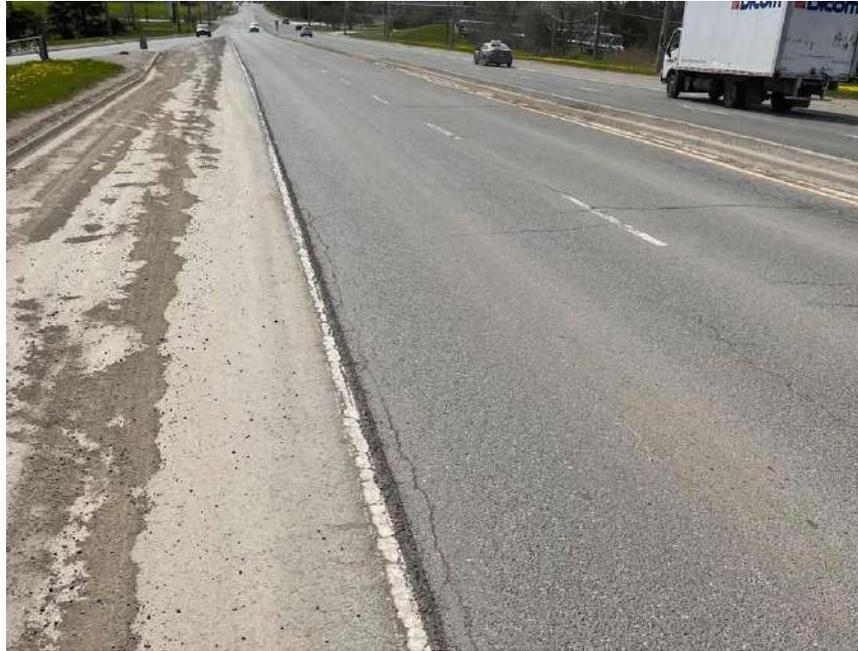
**Photograph 101 – Bramalea Road, Northbound, looking South, near East-South ramp of Highway 407, showing moderate longitudinal and transverse cracking associated with moderate random cracking, moderate pavement edge cracking and slight to moderate pavement raveling.**
