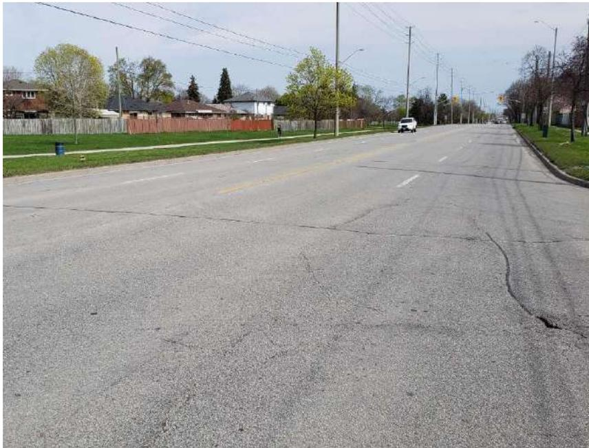
**Photograph 58 – Bramalea Road, Southbound, looking South, near the intersection of Bramalea Road and Algonquin Boulevard, showing moderate longitudinal and transverse cracking associated with slight to moderate random cracking and slight to moderate pavement raveling.**
