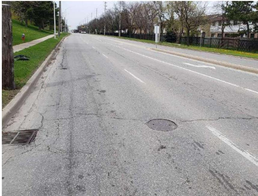
**Photograph 24 – Bramalea Road, Southbound, looking North, near the intersection of Bramalea Road and Clark Boulevard, showing moderate longitudinal and transverse cracking associated with slight to moderate random cracking, slight to moderate alligator cracking, slight to moderate pavement raveling and moderate to severe pavement edge cracking. Noting moderate to severe alligator cracking around catch basin.**
