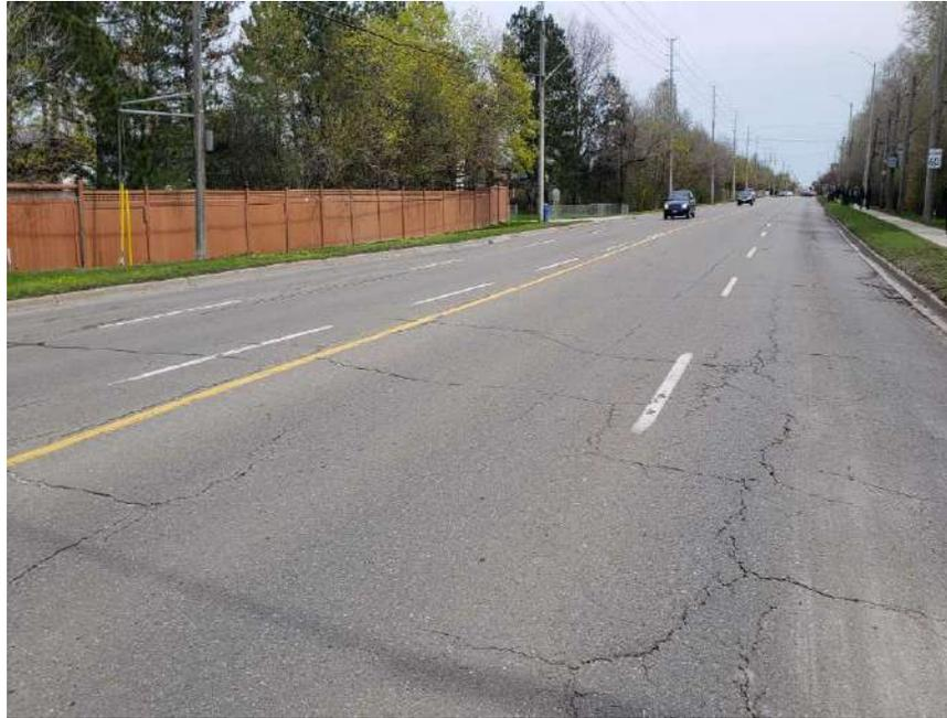
**Photograph 31 – Bramalea Road, Southbound, looking South, approximately 130 m South of Clark Boulevard, showing severe longitudinal and transverse cracking associated with moderate block cracking, moderate random cracking, slight pavement raveling, slight pavement depressions, slight alligator cracking and moderate pavement edge cracking.**
