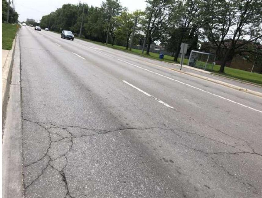
**Photograph 27 – Bramalea Road, Northbound, looking South, near the intersection of Bramalea Road and Clark Boulevard, showing slight to moderate longitudinal and transverse cracking associated with moderate random cracking, slight to moderate alligator cracking, slight pavement raveling and slight to moderate pavement edge cracking.**
