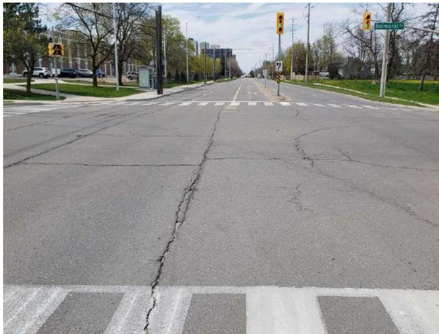
**Photograph 50 – Bramalea Road, looking North, near the intersection of Bramalea Road and Balmoral Drive, showing severe longitudinal and transverse cracking associated with moderate random cracking, slight alligator cracking and slight pavement raveling.**
