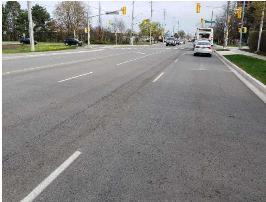
**Photograph 72 – Bramalea Road, Southbound, looking South, near the intersection of Bramalea Road and Avondale Boulevard, showing slight longitudinal cracking associated with slight random cracking.**
