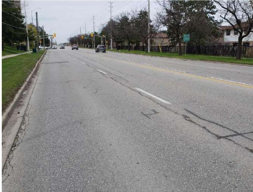
**Photograph 17 – Bramalea Road, Southbound, looking North, approximately 105 m South of Fleetwood Crescent, showing moderate longitudinal and transverse cracking associated with slight to moderate random cracking, slight pavement raveling, slight alligator cracking and moderate pavement edge cracking.**
