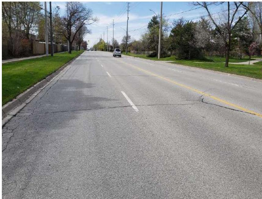
**Photograph 64 – Bramalea Road, Southbound, looking North, approximately 40 m North of Alexandria Gate, showing moderate longitudinal and transverse cracking associated with slight to moderate random cracking, slight to moderate pavement raveling, moderate to severe alligator cracking, and moderate to severe pavement edge cracking.**
