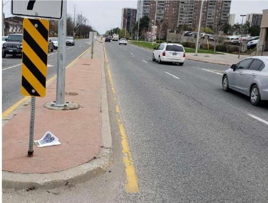
**Photograph 3 – Bramalea Road, Southbound, looking South, near the intersection of Queen Street East and Bramalea Road, showing moderate longitudinal and transverse cracking associated with slight to moderate random cracking, slight alligator cracking and slight pavement raveling.**
