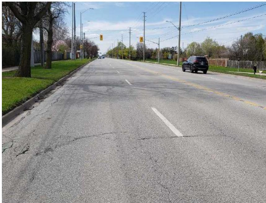
**Photograph 62 – Bramalea Road, Southbound, looking North, approximately 150 m North of Alexandria Gate, showing moderate longitudinal and transverse cracking associated with moderate random cracking, moderate pavement raveling, moderate alligator cracking and moderate to severe pavement edge cracking.**
