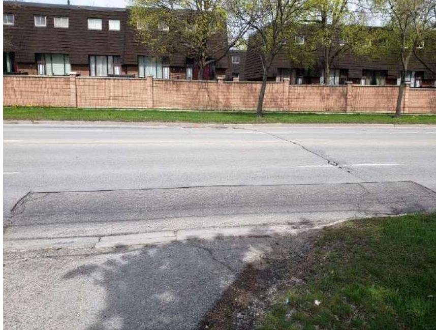
**Photograph 55 – Bramalea Road, Southbound, looking East, approximately 145 m South of Balmoral Drive, showing moderate longitudinal and transverse cracking associated with slight to moderate random cracking, slight pavement raveling, and moderate pavement edge cracking. Noting severe alligator cracking around catch basin and sections of patching.**
