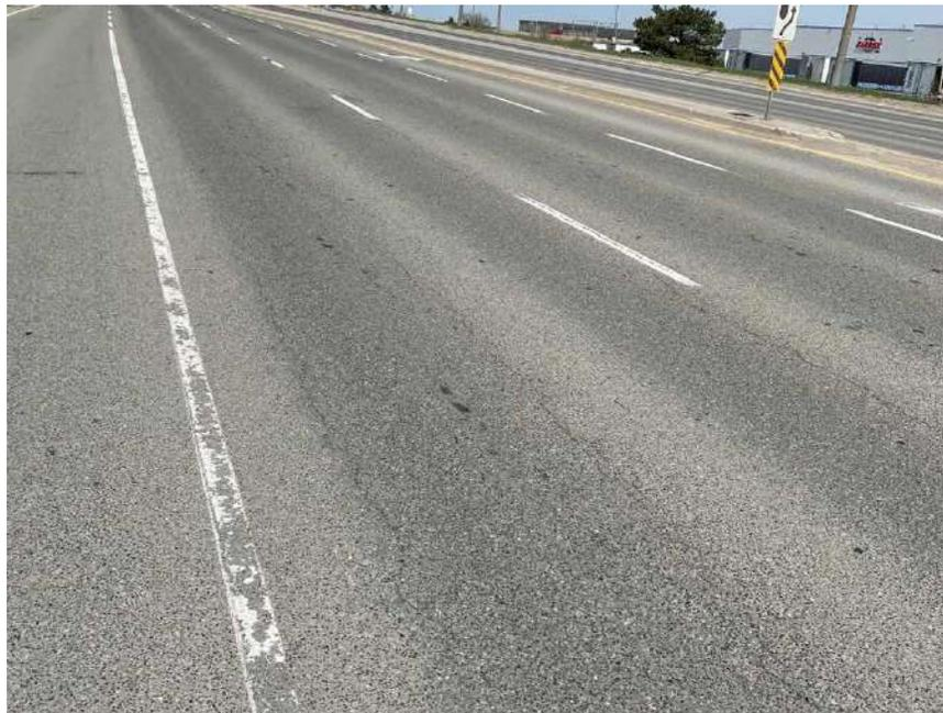
**Photograph 104 – Bramalea Road, Southbound, looking North, approximately 320 m South of Highway 407, showing slight to moderate longitudinal cracking associated with slight random cracking and slight to moderate pavement raveling.**
