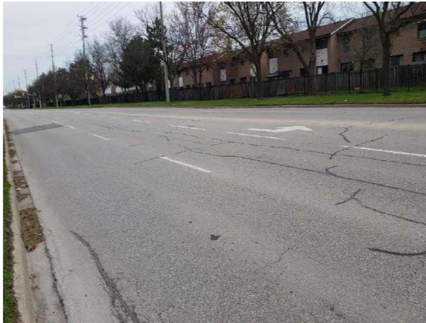
**Photograph 22 – Bramalea Road, Southbound, looking North, approximately 75 m North of Clark Boulevard, showing moderate to severe longitudinal and transverse cracking associated with moderate random cracking, slight block cracking, slight to moderate pavement raveling, and slight to moderate pavement edge cracking. Noting patching around catch basin and manhole.**
