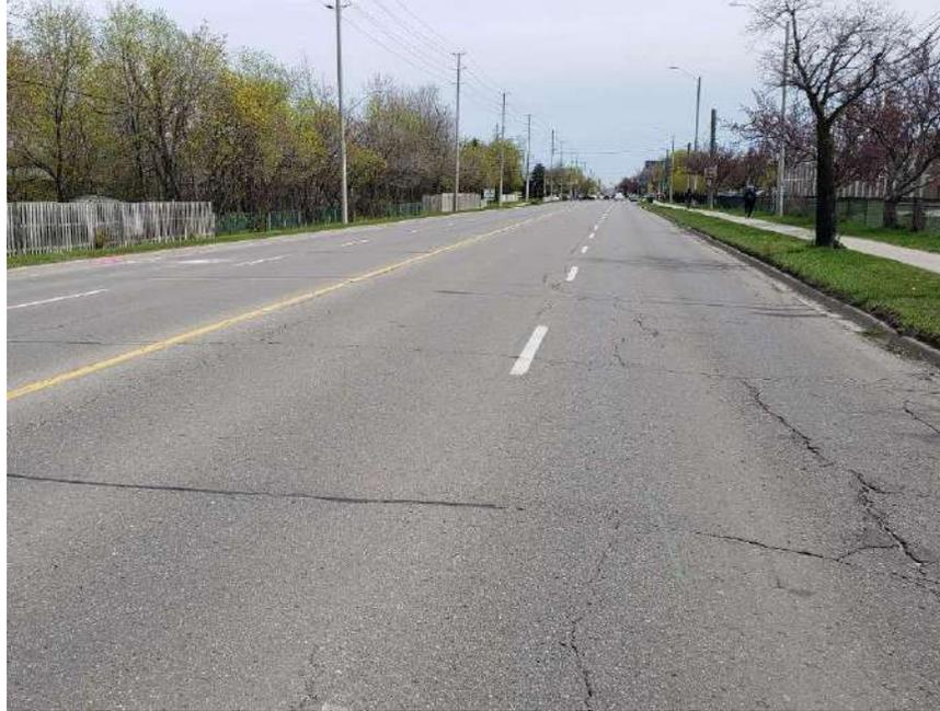
**Photograph 41 – Bramalea Road, Southbound, looking South, approximately 305 m North of Balmoral Drive, showing moderate to severe longitudinal and transverse cracking associated with moderate random cracking, slight alligator cracking, slight pavement raveling and slight to moderate pavement edge cracking.**
