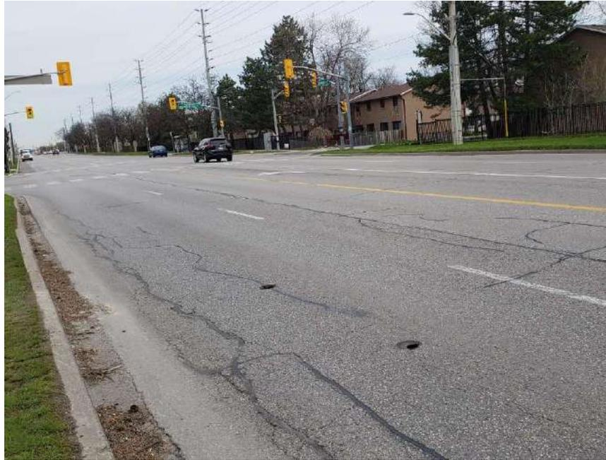
**Photograph 15 – Bramalea Road, Southbound, looking North, in the vicinity of the intersection of Bramalea Road and Fleetwood Crescent, showing moderate to severe longitudinal and transverse cracking associated with moderate random cracking, slight potholes, slight to moderate pavement raveling and moderate pavement edge cracking.**
