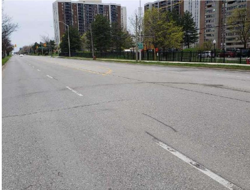
**Photograph 11 – Bramalea Road, Northbound, looking South, near the South intersection of Gates of Bramalea and Bramalea Road, showing slight to moderate longitudinal and transverse cracking associated with slight random cracking, slight pavement edge cracking and slight pavement raveling. Noting sections of patching.**
