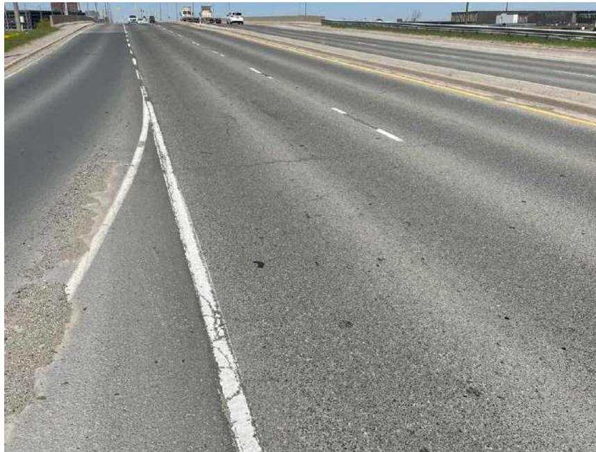
**Photograph 100 – Bramalea Road, Southbound, looking North, near West-South Ramp of Highway 407, showing slight longitudinal and transverse cracking associated with slight to moderate random cracking, slight alligator cracking, and moderate pavement raveling.**
