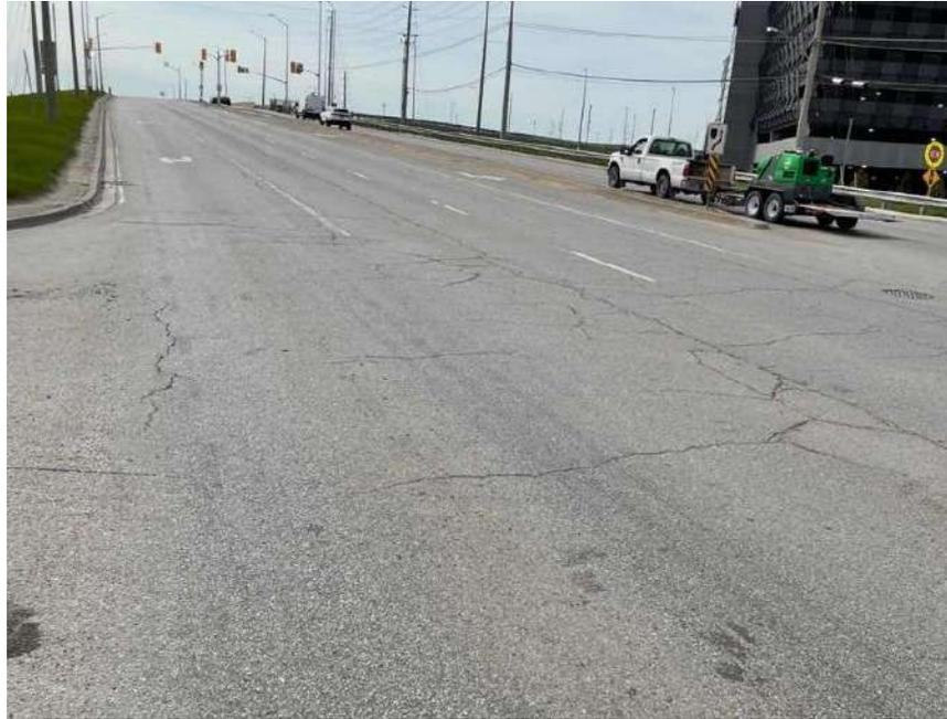
**Photograph 85 – Bramalea Road, Northbound, looking South, approximately 120 m South of Steeles Avenue East, showing moderate to severe longitudinal and transverse cracking associated with moderate to severe random cracking, moderate to severe block cracking and slight pavement raveling.**
