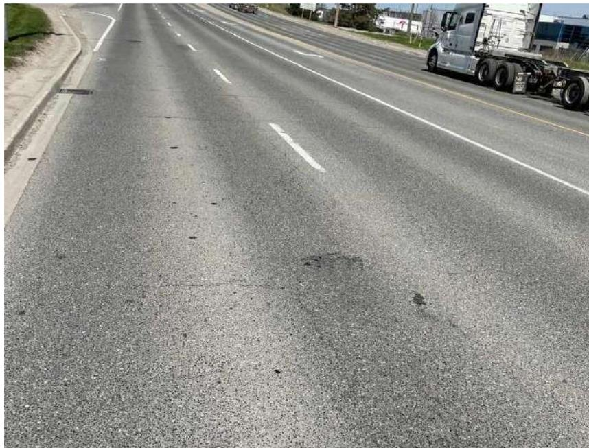
**Photograph 106 – Bramalea Road, Southbound, looking North, approximately 420 m South of Highway 407, showing moderate longitudinal and transverse cracking associated with slight to moderate random cracking and slight to moderate pavement raveling.**
