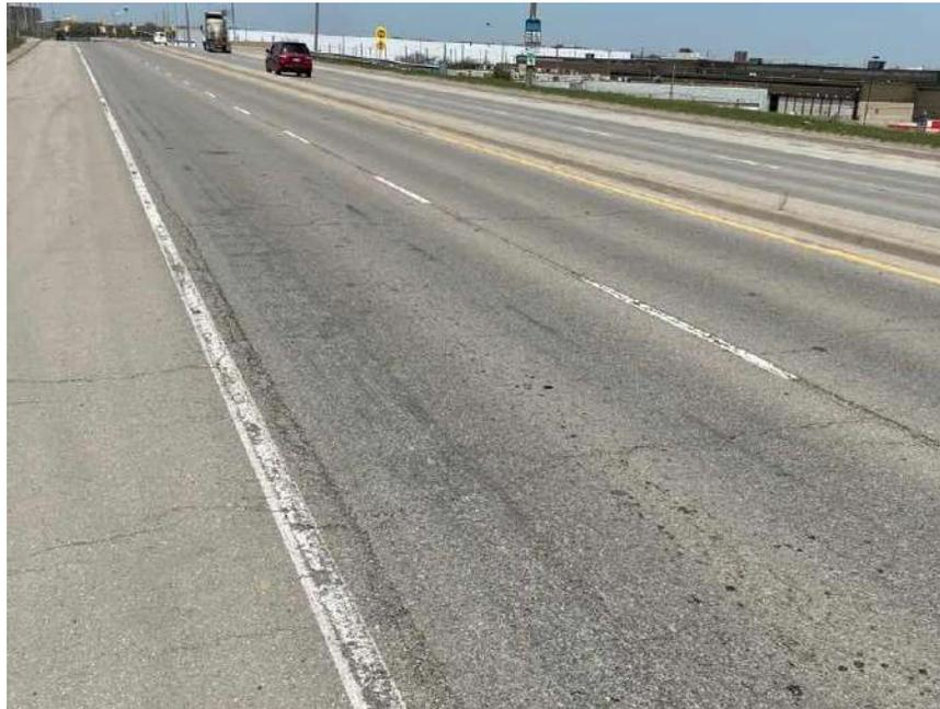
**Photograph 96 – Bramalea Road, Southbound, looking North, approximately 170 m South of Railway, showing moderate to severe longitudinal and transverse cracking associated with moderate random cracking, moderate pavement raveling, slight block cracking and slight alligator cracking.**
