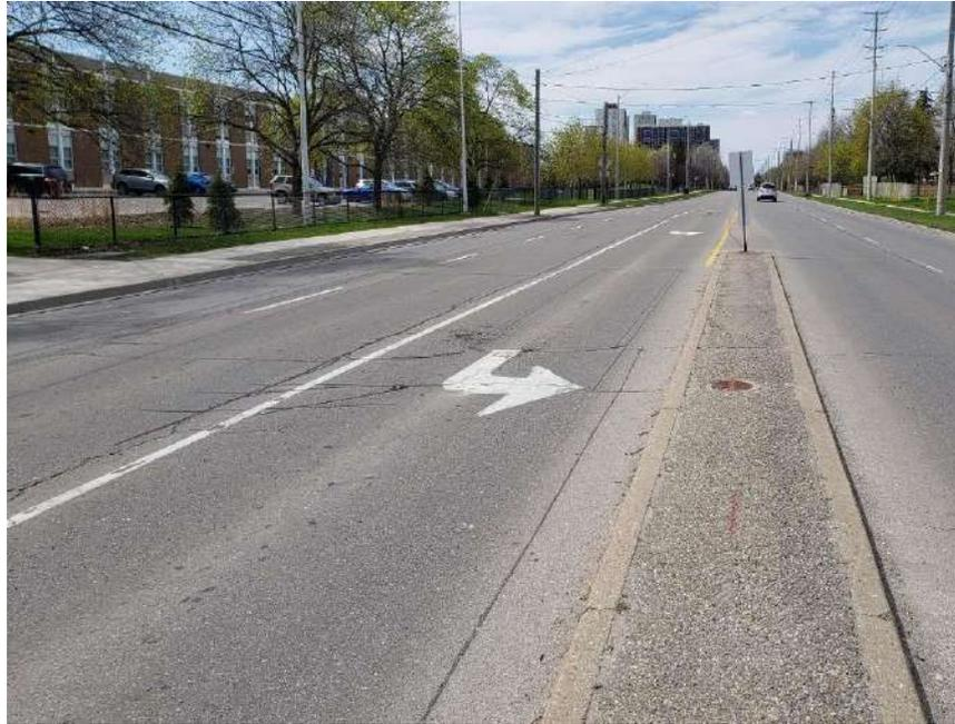
**Photograph 49 – Bramalea Road, Southbound, looking North, near the intersection of Bramalea Road and Balmoral Drive, showing moderate to severe longitudinal and transverse cracking associated with moderate random cracking, moderate block cracking, slight to moderate potholes and slight pavement raveling.**
