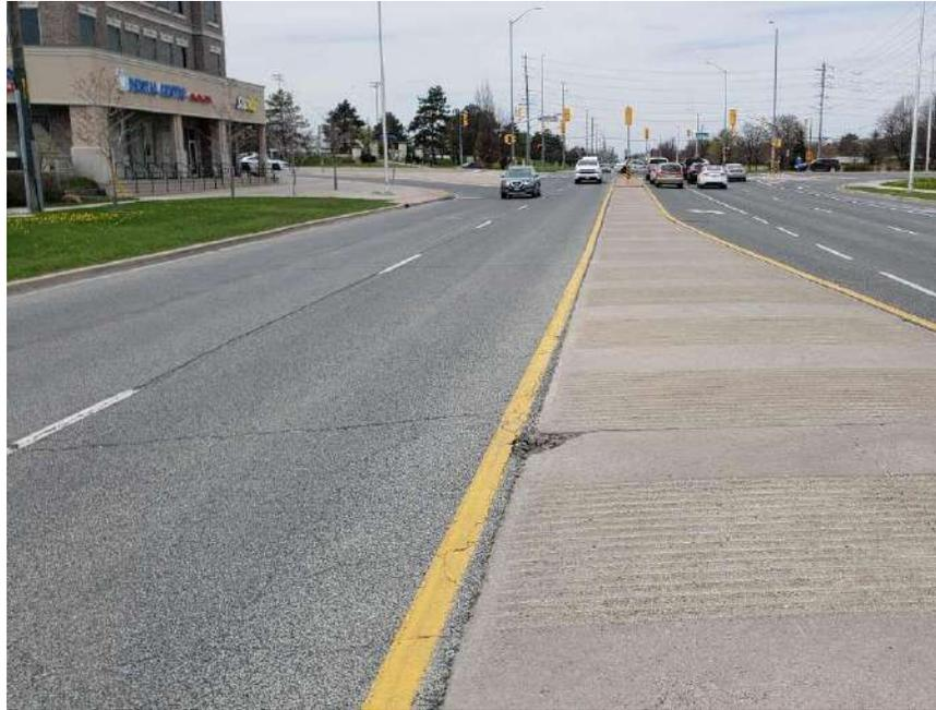
**Photograph 5 – Bramalea Road, Southbound, looking North, approximately 110 m South of Queen Street East, showing moderate longitudinal and transverse cracking associated with slight to moderate random cracking, slight potholes, slight pavement edge cracking and slight pavement raveling.**
