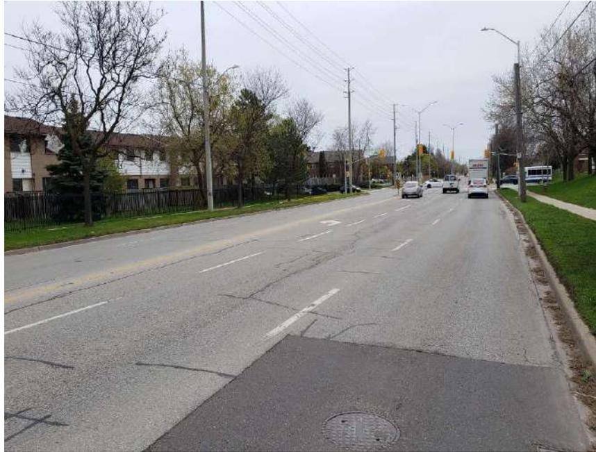
**Photograph 21 – Bramalea Road, Southbound, looking South, approximately 100 m North of Clark Boulevard, showing moderate to severe longitudinal and transverse cracking associated with slight to moderate random cracking, slight to moderate pavement raveling and slight pavement edge cracking. Noting patching around catch basin and manhole.**
