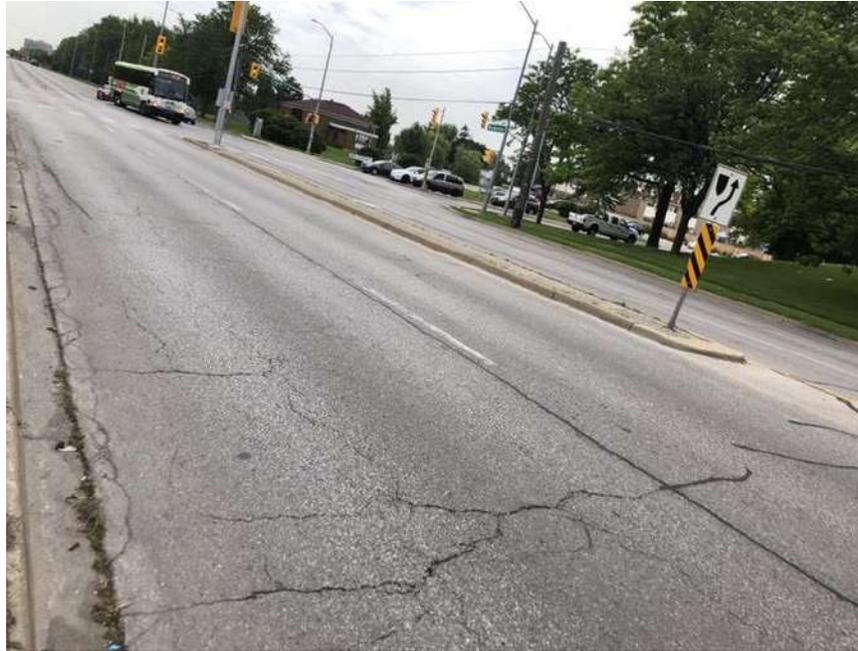
**Photograph 23 – Bramalea Road, Northbound, looking South, approximately 50 m North of Clark Boulevard, showing moderate to severe longitudinal and transverse cracking associated with moderate to severe random cracking, slight alligator cracking, slight pavement raveling and moderate to severe pavement edge cracking.**
