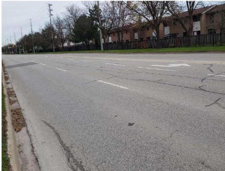
**Photograph 18 – Bramalea Road, Southbound, looking North, approximately 125 m South of Fleetwood Crescent, showing moderate to severe longitudinal and transverse cracking associated with moderate random cracking, slight to moderate pavement raveling and slight to moderate pavement edge cracking.**
