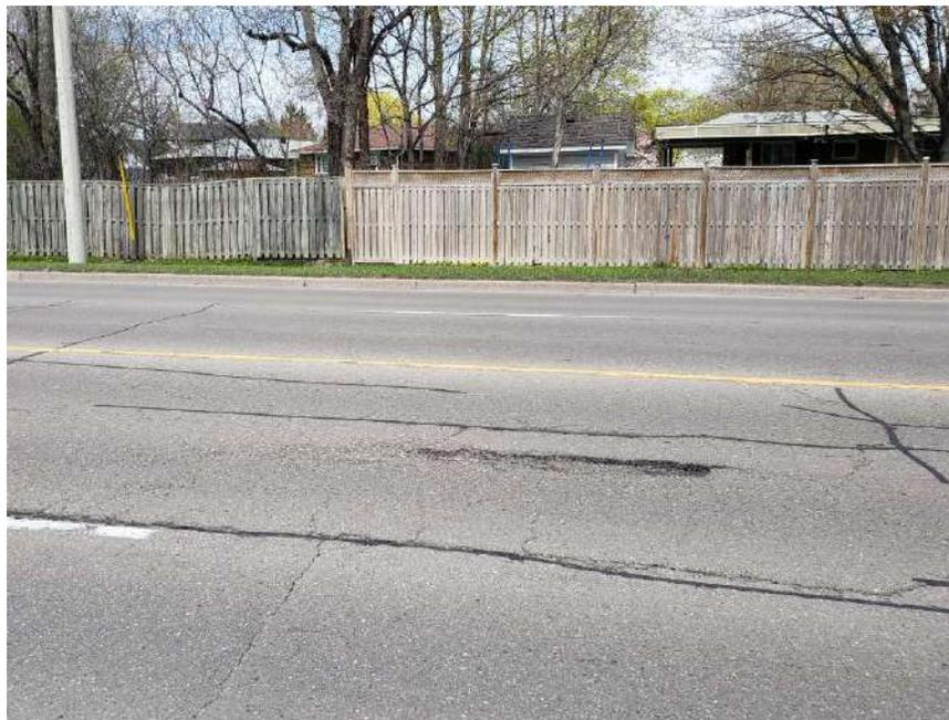
**Photograph 44 – Bramalea Road, Southbound, looking East, approximately 205 m North of Balmoral Drive, showing severe longitudinal and transverse cracking associated with moderate random cracking, slight to moderate potholes and slight pavement raveling.**
