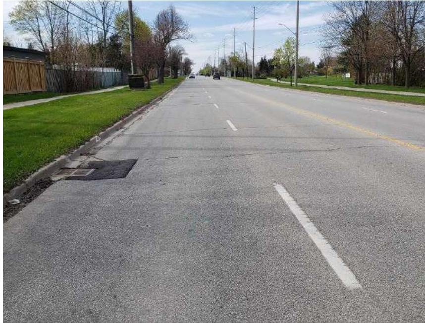
**Photograph 69 – Bramalea Road, Southbound, looking North, approximately 170 m South of Alexandria Gate, showing moderate longitudinal and transverse cracking associated with slight random cracking, slight to moderate pavement raveling and moderate pavement edge cracking. Noting patching around catch basin.**
