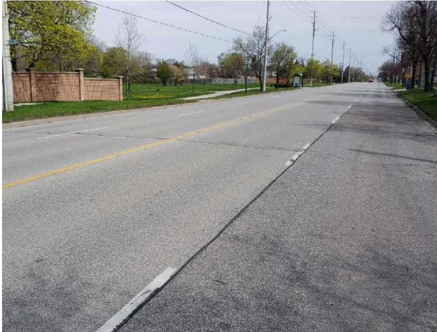
**Photograph 57 – Bramalea Road, Southbound, looking South, near the intersection of Bramalea Road and Darras Court, showing moderate longitudinal and transverse cracking associated with slight random cracking, slight to moderate pavement raveling and slight pavement edge cracking. Noting severe alligator cracking around catch basin and sections of patching.**
