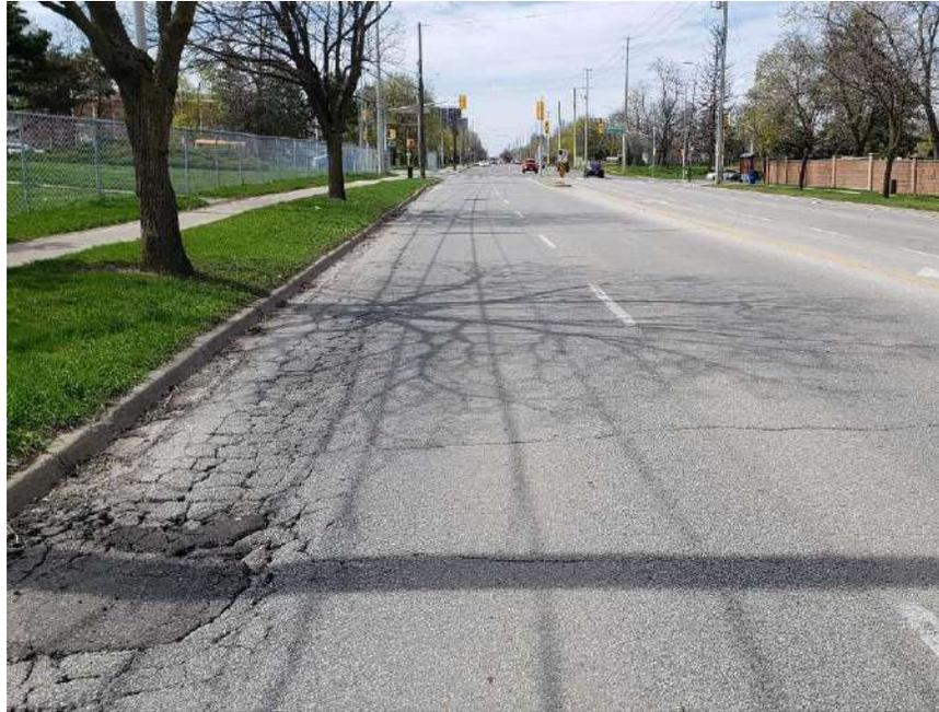
**Photograph 53 – Bramalea Road, Southbound, looking North, approximately 95 m South of Balmoral Drive, showing slight to moderate longitudinal and transverse cracking associated with severe alligator cracking, moderate pavement depressions, slight to moderate pavement raveling, slight pavement patching, and moderate to severe pavement edge cracking.**
