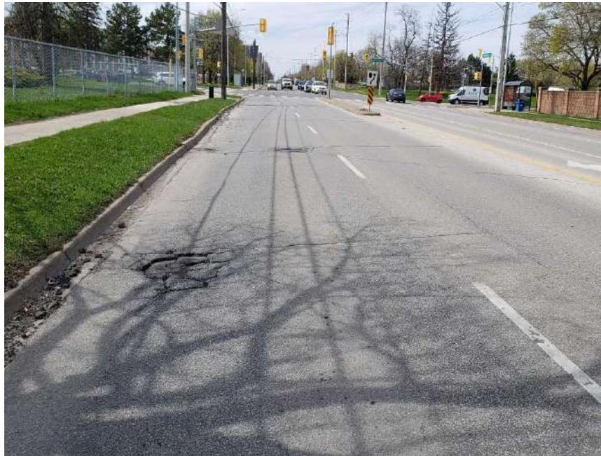
**Photograph 52 – Bramalea Road, Southbound, looking North, approximately 70 m South of Balmoral Drive, showing moderate longitudinal and transverse cracking associated with moderate random cracking, severe alligator cracking, slight to moderate pavement raveling, slight to moderate potholes and severe pavement edge cracking.**
