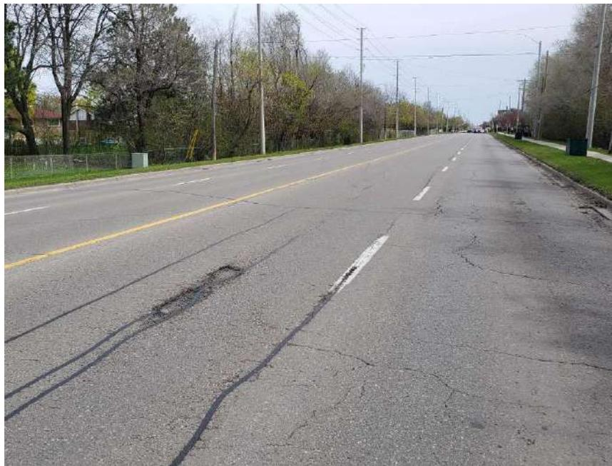
**Photograph 34 – Bramalea Road, Southbound, looking South, approximately 175 m South of Clark Boulevard, showing moderate to severe longitudinal and transverse cracking associated with moderate random cracking, slight pavement raveling, slight potholes and moderate pavement edge cracking.**
