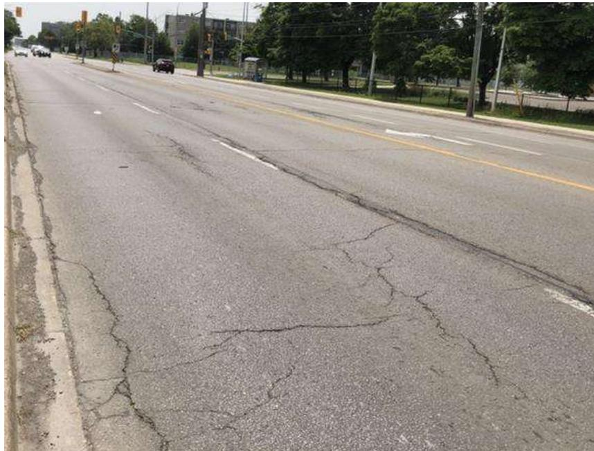
**Photograph 48 – Bramalea Road, Northbound, looking South, approximately 95 m North of Balmoral Drive, showing severe longitudinal and transverse cracking associated with moderate random cracking, slight pavement depressions, slight to moderate pavement raveling and moderate pavement edge cracking.**
