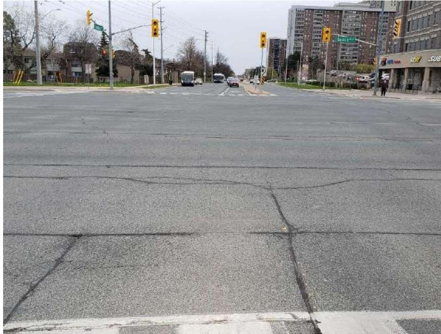
**Photograph 1 – Bramalea Road, looking South, near the intersection of Queen Street East and Bramalea Road, showing moderate to severe longitudinal and transverse cracking associated with slight to moderate random cracking and slight pavement raveling.**
