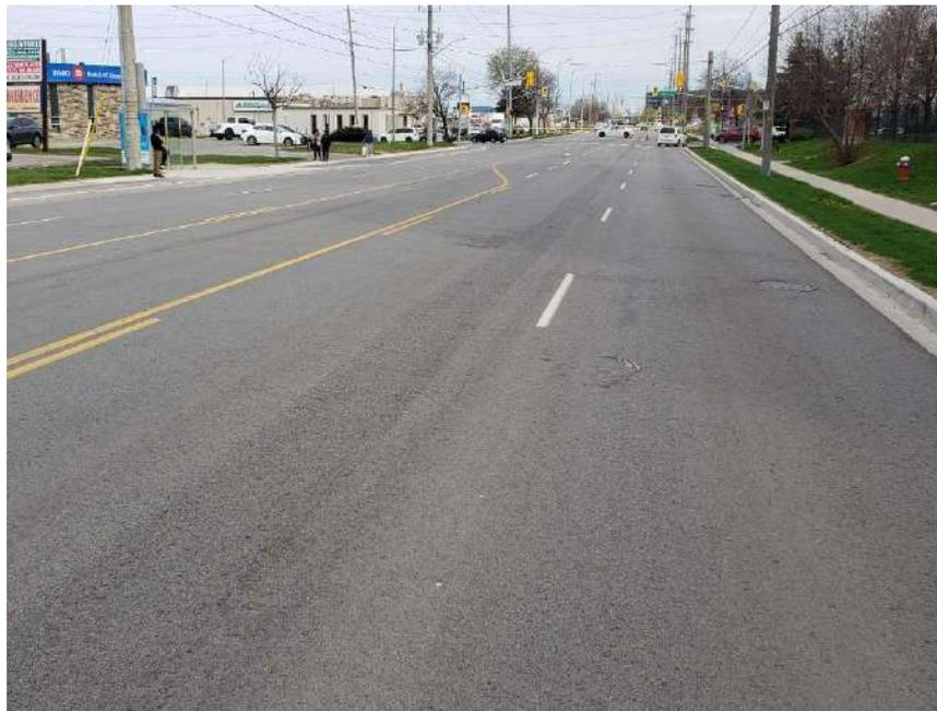
**Photograph 76 – Bramalea Road, Southbound, looking South, approximately 75 m north of East Drive, showing relatively newly paved asphalt concrete.**
