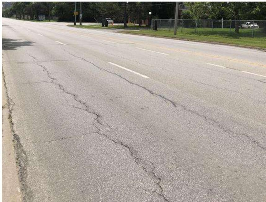
**Photograph 54 – Bramalea Road, Northbound, looking South, approximately 100 m South of Bramalea Road, showing severe longitudinal and transverse cracking associated with moderate random cracking, slight to moderate pavement raveling and slight to moderate pavement edge cracking.**
