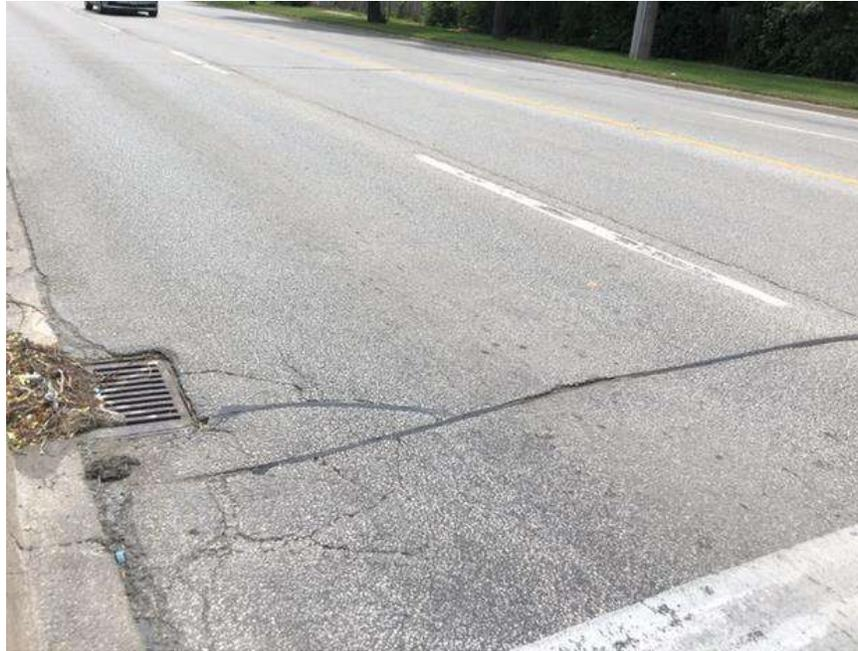
**Photograph 61 – Bramalea Road, Northbound, looking South, approximately 155 m South of Algonquin Boulevard, showing moderate longitudinal and transverse cracking associated with slight to moderate random cracking, slight to moderate pavement raveling and slight to moderate pavement edge cracking. Noting severe random cracking around catch basin.**
