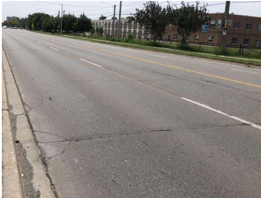
**Photograph 42 – Bramalea Road, Northbound, looking South, approximately 235 m North of Balmoral Drive, showing moderate to severe longitudinal and transverse cracking associated with slight to moderate random cracking, slight pavement raveling and slight to moderate pavement edge cracking.**
