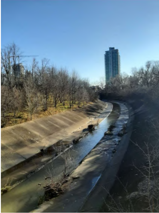
Photograph 13: Etobicoke Creek, north of the Site.
