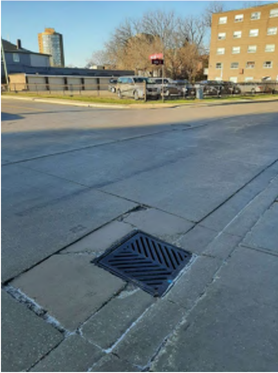
Photograph 7: On-site catch basins located at south entrance of the Site.
