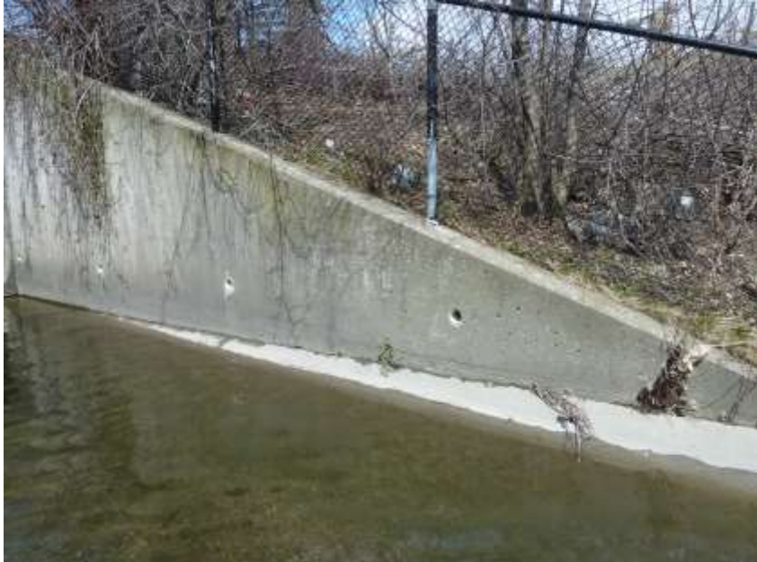
PHOTOGRAPH 3 OUT END WALL - NORTH
