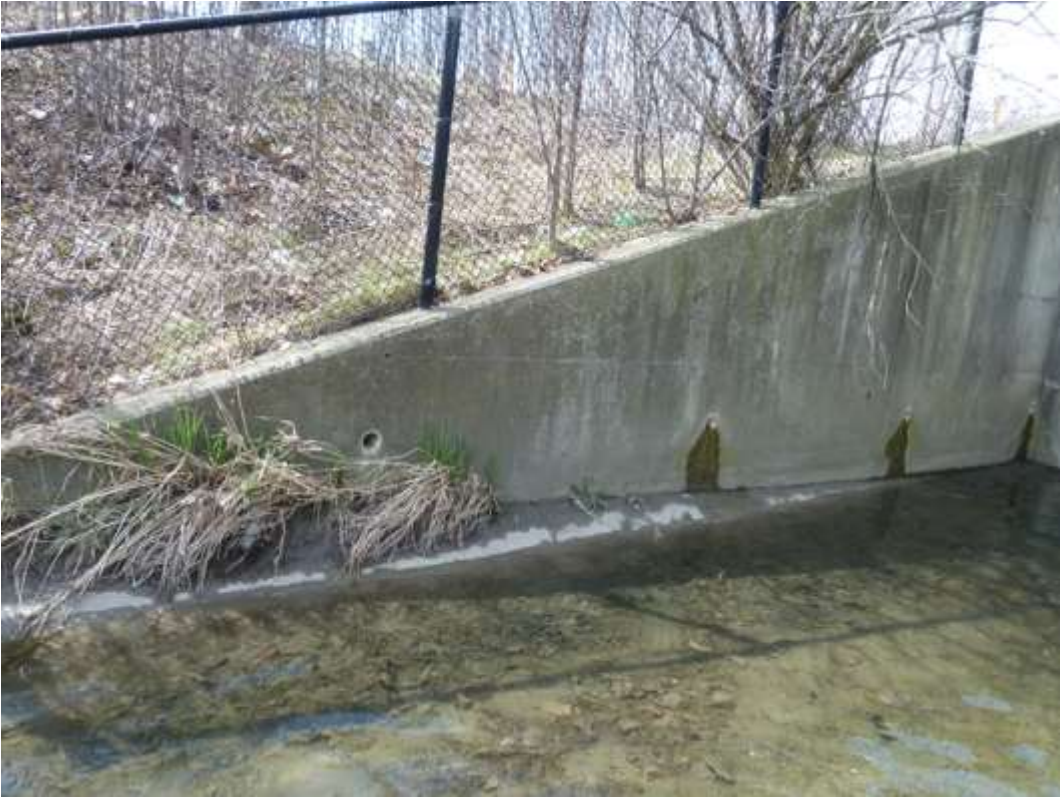
PHOTOGRAPH 2 OUTLET END WALL - SOUTH
