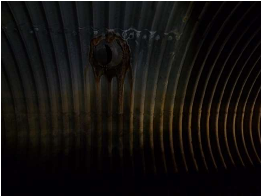
PHOTOGRAPH 8 CULVERT BARREL - RUSTED
