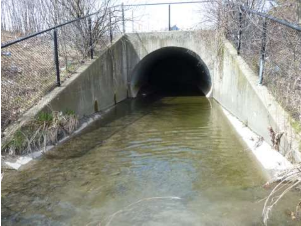
PHOTOGRAPH 1 OUTLET END WALLS
