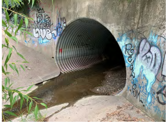
Photo 12: View of Mimico Creek culvert from upstream, facing north.
