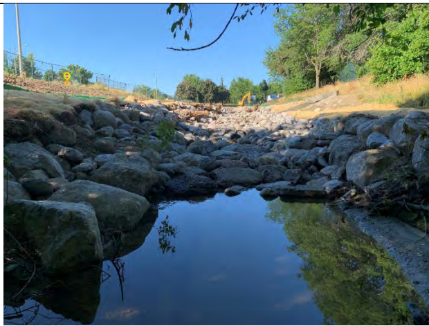
Photo 7: View of reconstructed Mimico Creek and area of restoration by TRCA.
