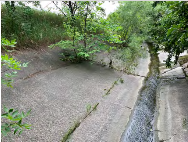
Photo 13: View from culvert of upstream Mimico Creek, facing south.
