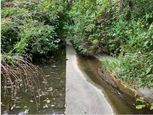
Photo 15: View of upstream Mimico Creek pool adjacent to concrete lining, facing south.
