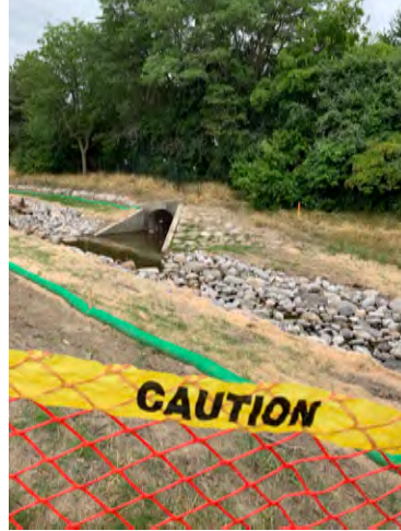
Photo 16: View of drainage culvert discharging into Mimico Creek within TRCA restoration area, facing east.
