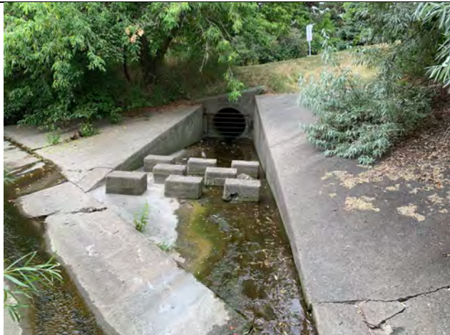
Photo 14: View of drainage culvert discharging into Mimico Creek, facing east.
