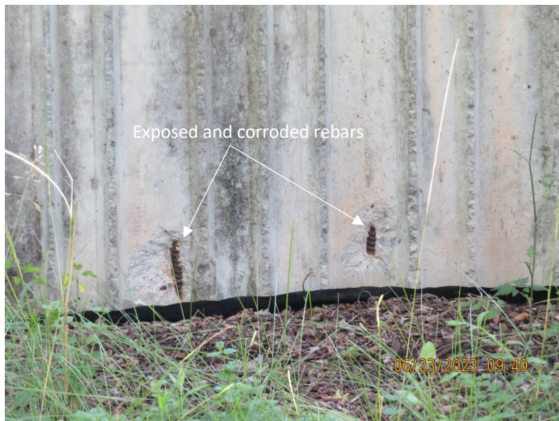
Photo 2-5: Exposed and corroded rebar
