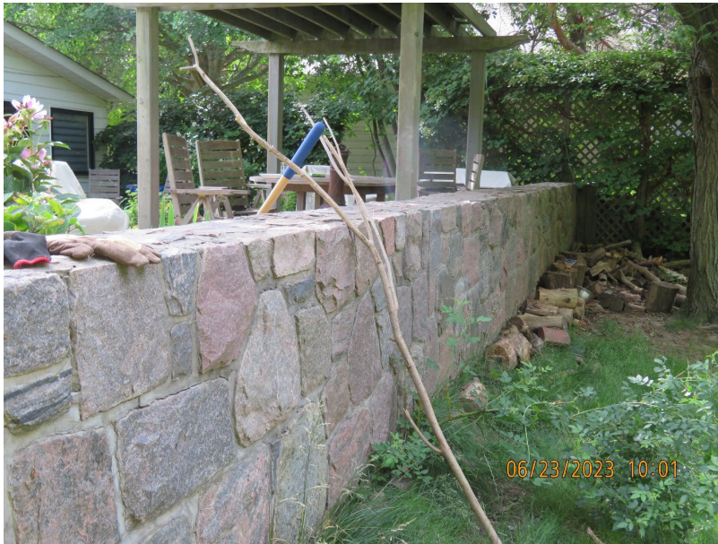
Photo 2-11: Floodwall section with stone cladding surface finish
