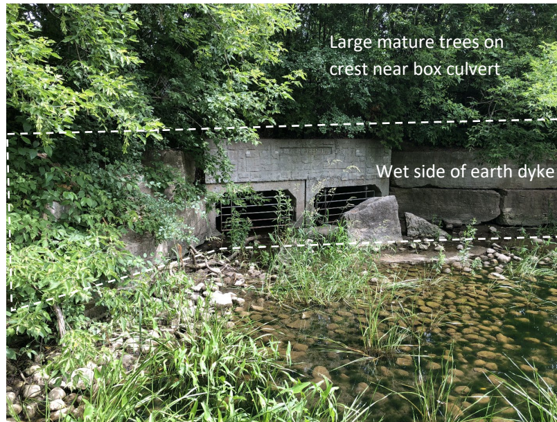
Photo 2-25: Stormwater box culvert outlet (OF_3977 and OF_3978)
