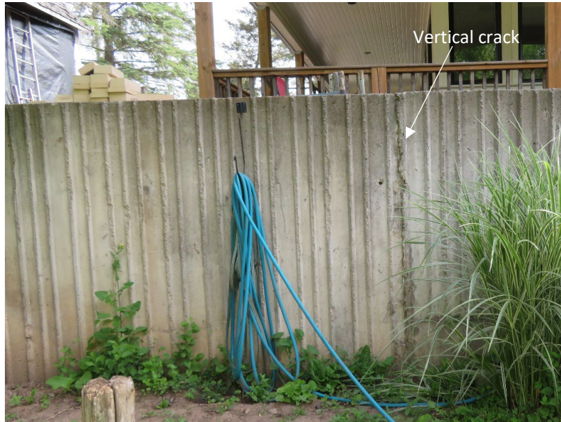
Photo 2-4: Vertical crack in concrete wall
