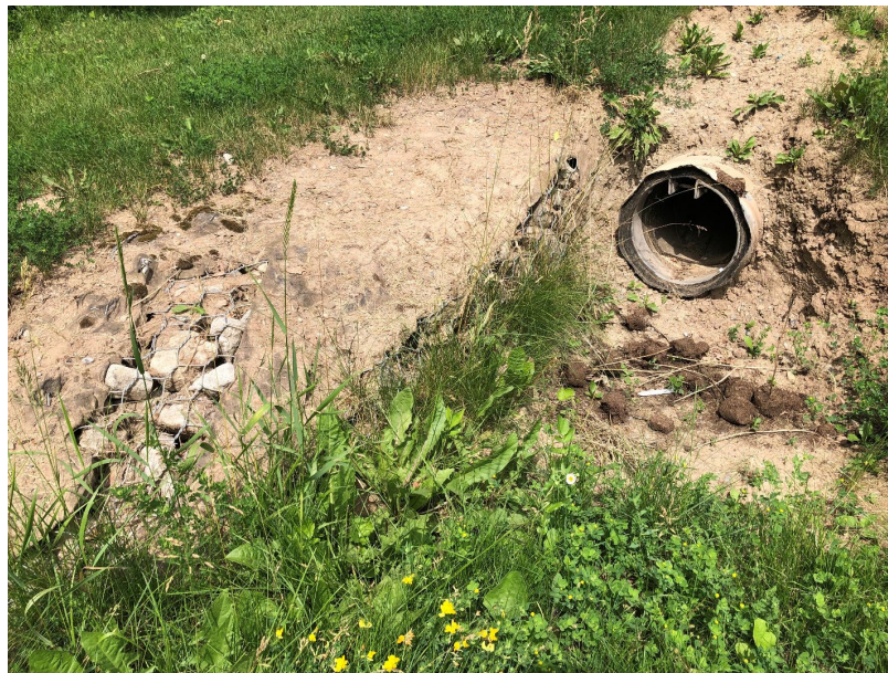
Photo 2-26: CSP culvert with inline check valve (OF_3979) near corner of Martins Blvd and Victoria Street
