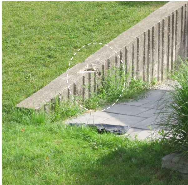
Photo 2-10: Crack in floodwall at wet-side toe
