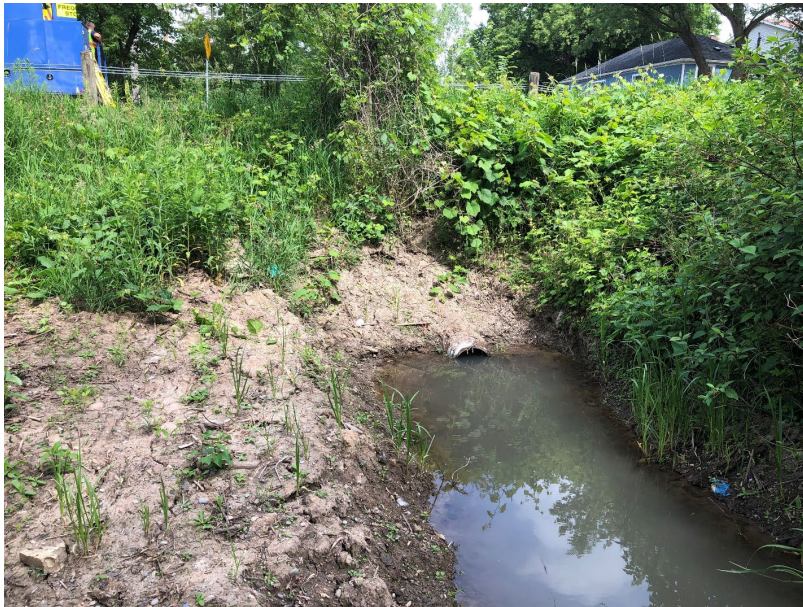
Photo 2-29: CSP culvert with inline check valve (OF_3980) at end of earth dyke section along Martins Blvd
