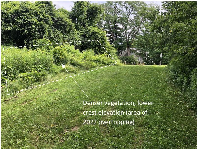
Photo 2-24: Wet side slope of dyke at Segment 4, near box culvert (area of 2022 overtopping)
