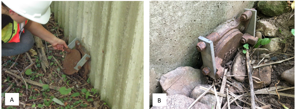
Photo 2-6: (a) Flap gate at northwest corner of floodwall segment (OF_3983) (b) Flap gate at southeast corner of floodwall with partial blockage (OF_3984)
